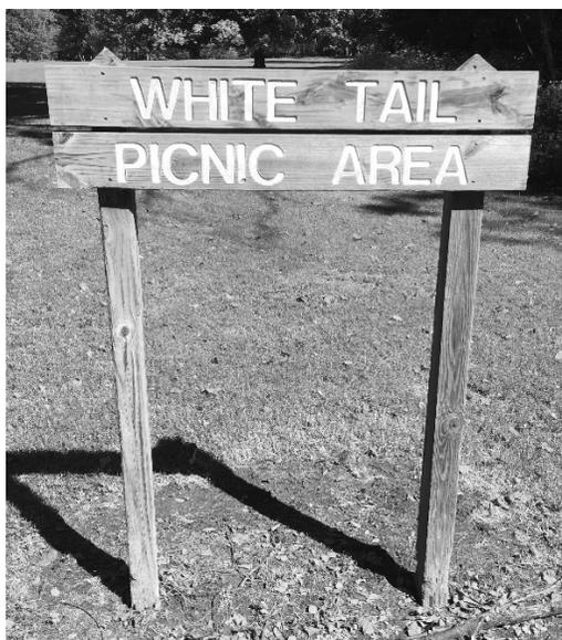
Sign support posts shall be 4 x 4 fiberglass reinforced recycled plastic lumber. All supports shall be straight and plumb, with a burry depth of 4'-0", and unless noted differently, shall be backfilled with porous granular material compacted around the support. The upper six inches of the backfill material shall be topsoil and shall be seeded with a Class 1A mixture.
