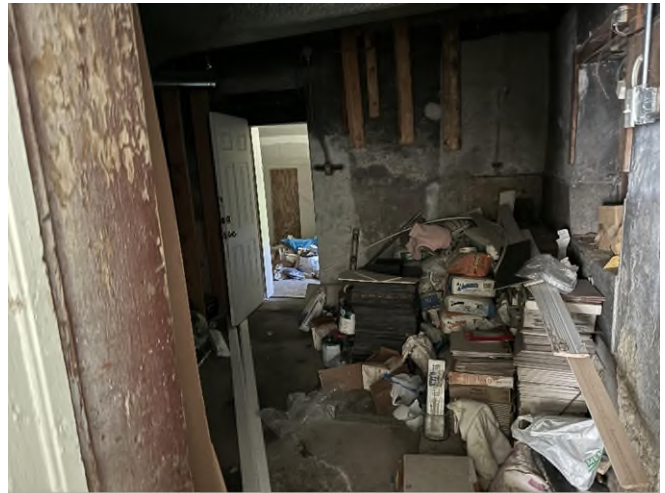
HA-14: Gray Concrete Foundation
