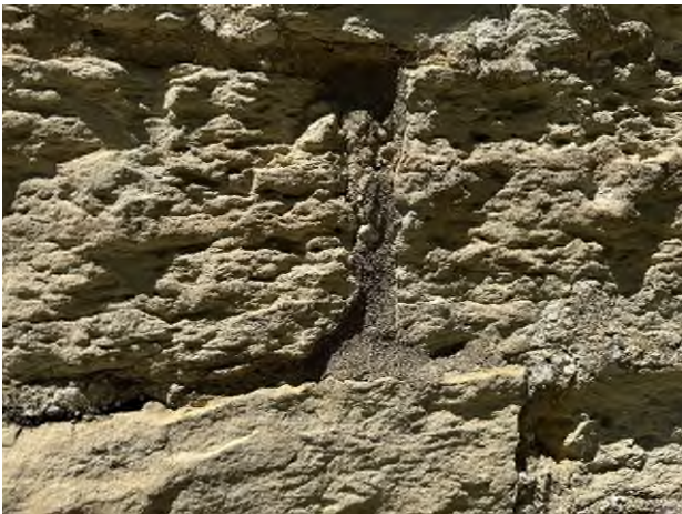
HA-22: Gray Mortar associated with Stone
