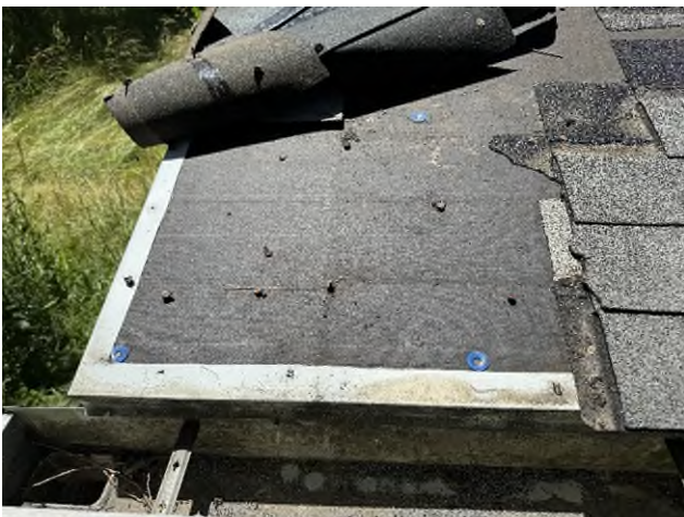
HA-15: Black Asphalt Shingles HA-16: Black Felt Layer under HA-15
