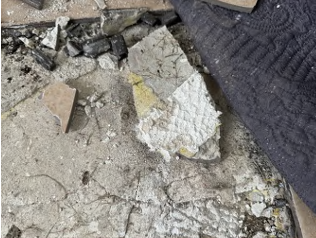
HA-10: Gray Leveling Compound under HA-5
