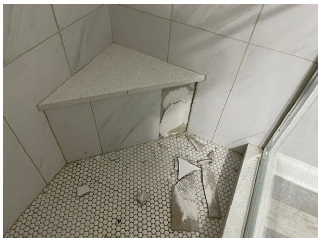
HA-4: White 1' x 3' Ceramic Wall Tile HA-5: White Adhesive associated with HA-4 HA-6: Gray Grout associated with HA-4
