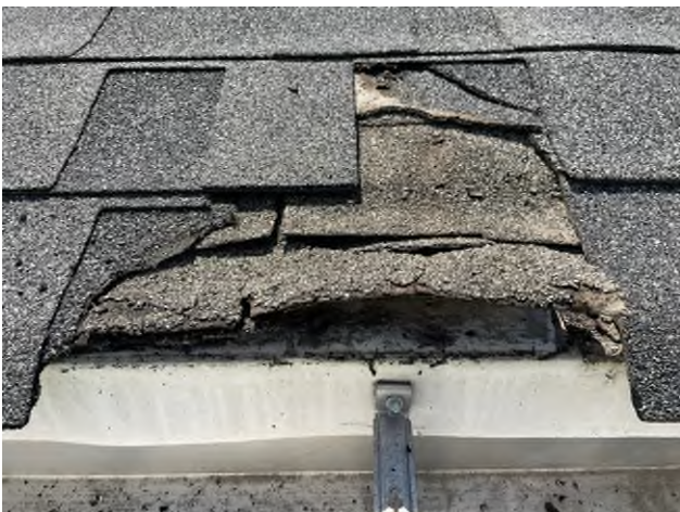
HA-25: Tar/Felt Roofing Paper beneath HA-24
