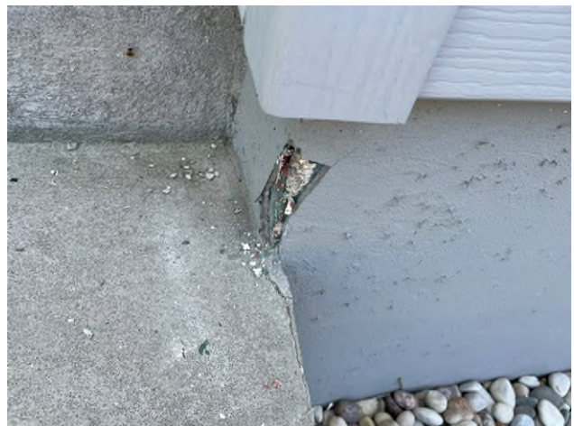
HA-26: Concrete Foundation
