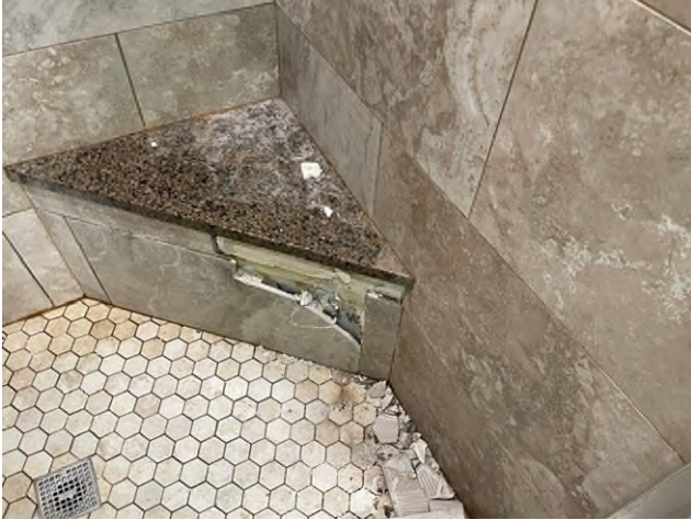
HA-19: Beige 1' x 2' Ceramic Wall Tile HA-20: White Adhesive associated with HA-19 HA-21: Dark Gray Grout associated with HA-19
