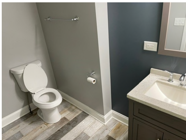
HA-1: Gypsum board
