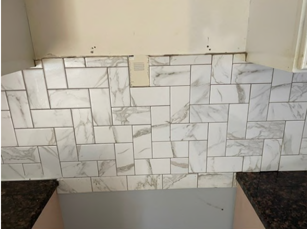
HA-27: White Ceramic Wall Tile Backsplash HA-28: Beige Adhesive associated with HA-27 HA-29: Brown Grout associated with HA-27
