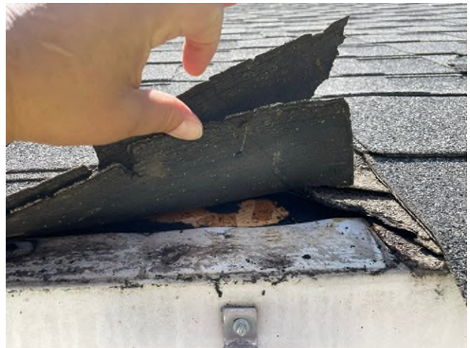
HA-24: Asphalt Roof Shingles
