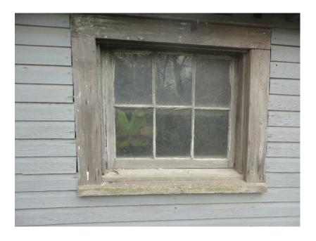
Material Description: Window Glazing, Grey – Tested Positive for Asbestos
