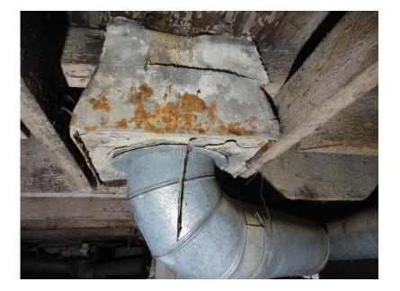
**Material Description:** Duct Tape, Grey, HVAC Duct Work - Tested Positive for Asbestos
