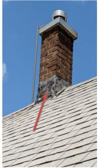
Material Description: Chimney and Exhaust Flashing - Tested Positive for Asbestos
