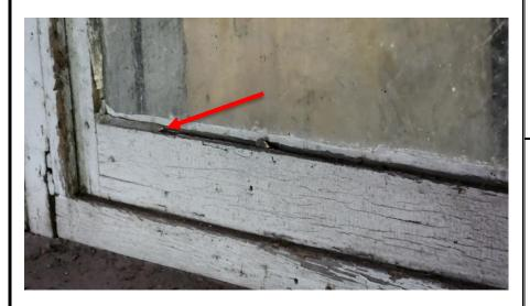
**Material Description:** Window Glazing - Tested **Positive for Asbestos**
