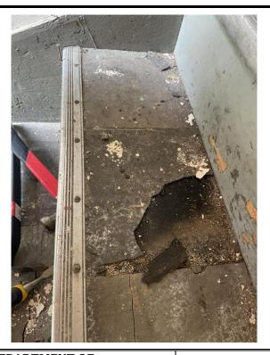
Material Description: 9"x9" Grey VFT & Black Mastic and 9"x9" Black VFT & Black Mastic – Tested Positive for Asbestos
