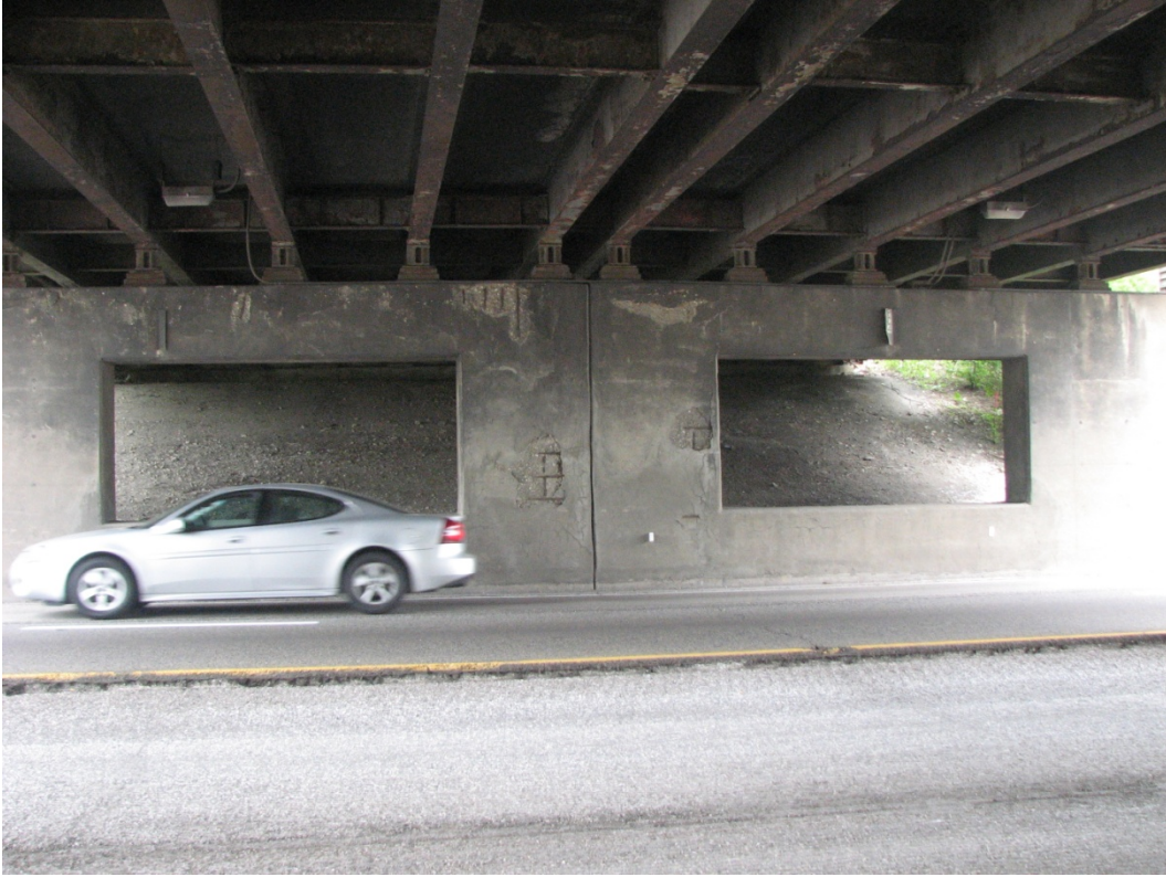
Photo 3 – Typical Pier and Underdeck Layout (Note Gravel Slopewall in Background)
