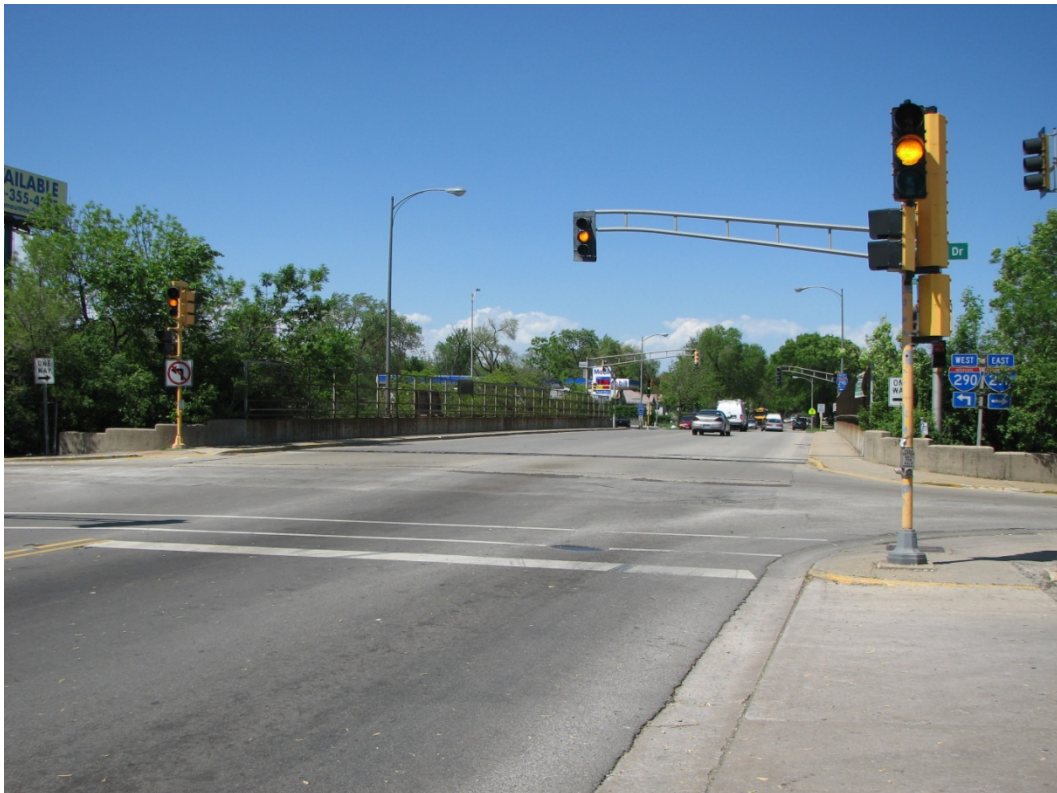
Photo 2 – Top of Bridge Looking North
