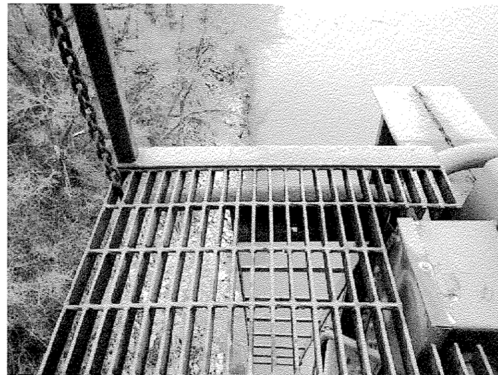
ITEM 677 Span 9, LOS (Catwalk) See Note A
