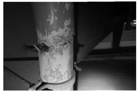
BROKEN FLOOR DRAIN EXTENSION PIPE
