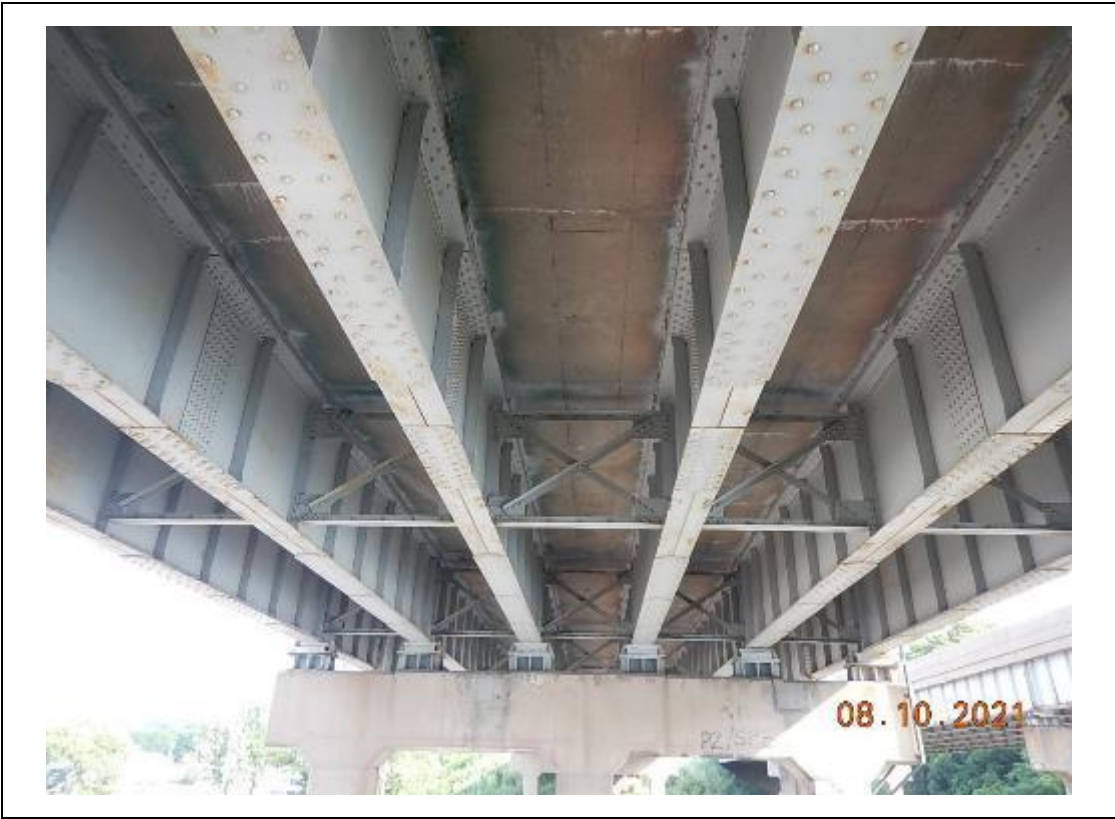
PHOTO 5 Span 3 looking North
