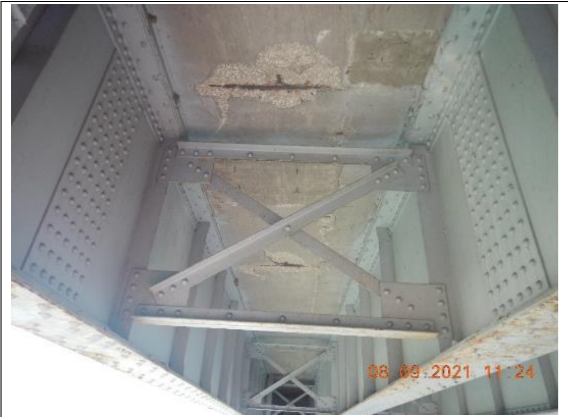
PHOTO 6 Span 7 looking South
