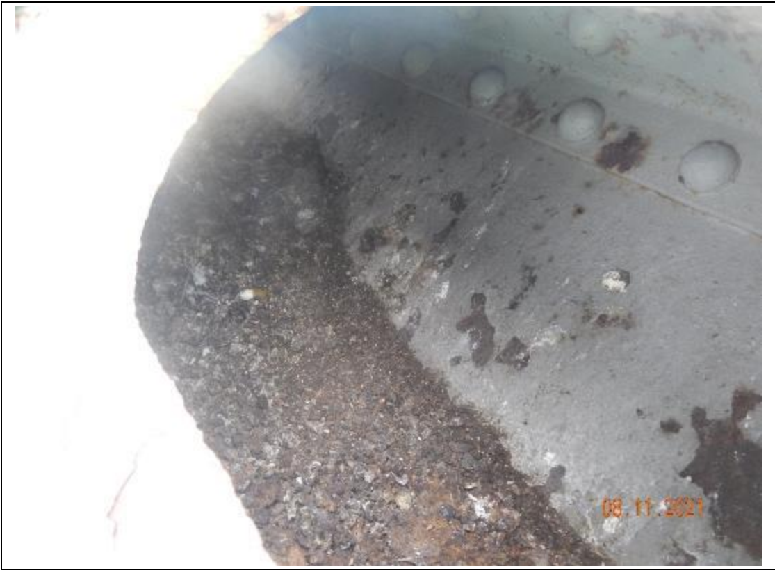
PHOTO 14 Span 6 looking Southeast
