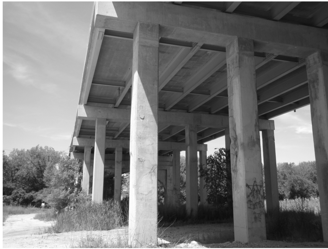
PIER 11 - LOOKING NORTH (Pier 13 & 17 similar)
