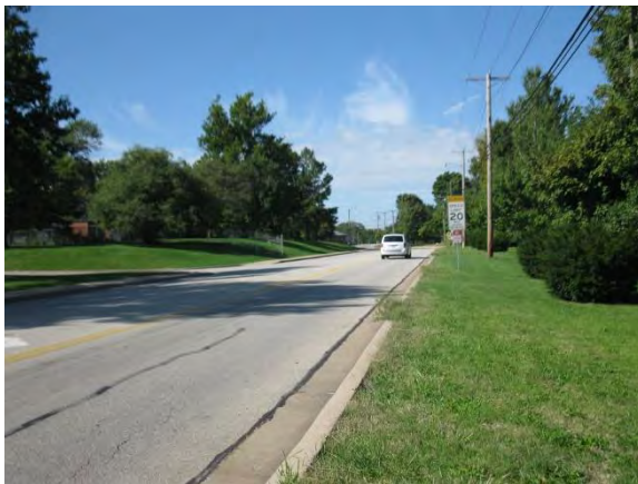
5. Looking west along West Grant Street.
