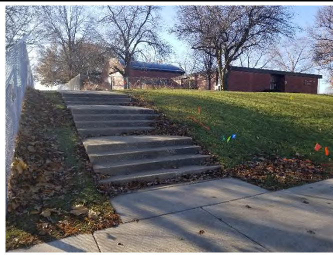
Photograph 4: View of north extent of Project Area, facing south
