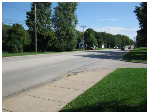
6. Looking east along West Grant Street.
