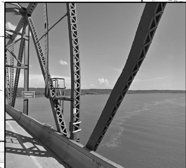
SAMPLE STEEL SECTION TO BE SALVAGED FOR PARK SCULPTURE
