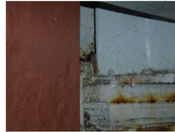
Picture 18: P22 BM9 BEAM END LOOKING S (R25)
