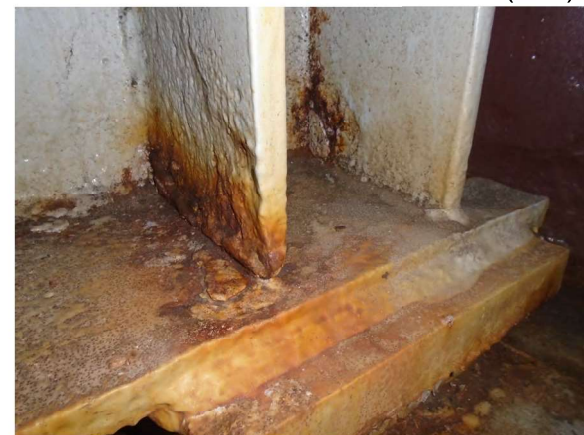
Picture 12: P21 WS SP 22 BM 15 SS LOOKING NE (R19)
