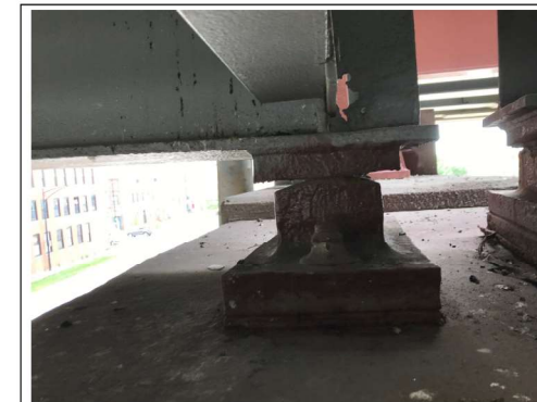
PHOTO #11 SPAN 10 BM GB-3 AT PIER B11 SS LKG W (R6)
