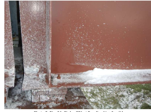
Photo 5: Pier 24, Girder G51 at Brg. (Looking South)
