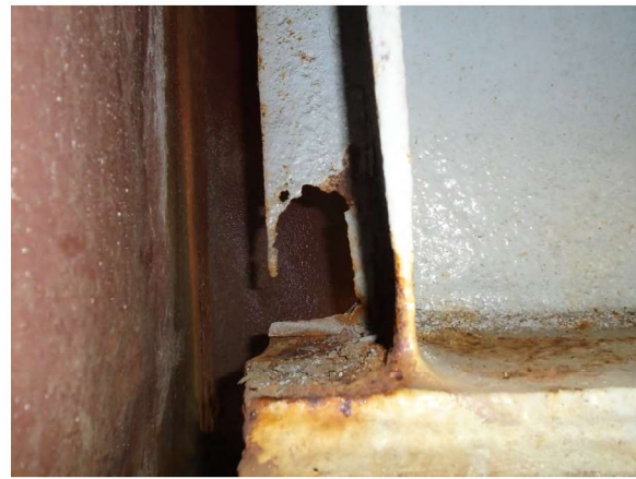
Picture 7: P19 WS SP 20 BM5 NS LOOKING S (R12)
