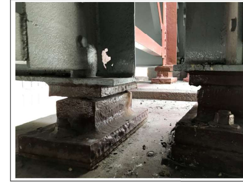
PHOTO #12 SPAN 10 BM GB-3 AT PIER B11 SS LKG SW (R6)
