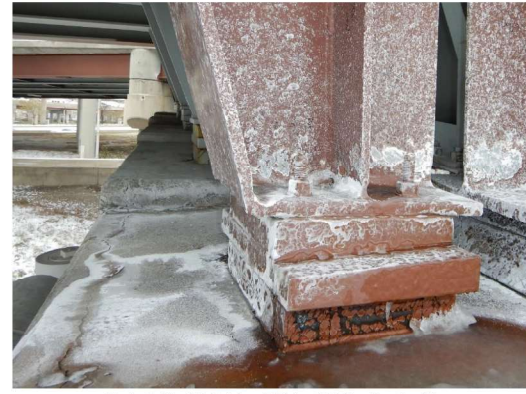
Photo 3: Pier 24, Bolster at Girder G57 (Looking South)
