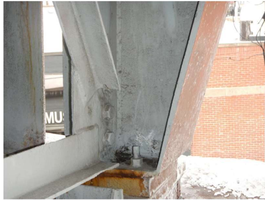
Photo 1: Pier 24, Bolster at Girder G57 (Looking North)
