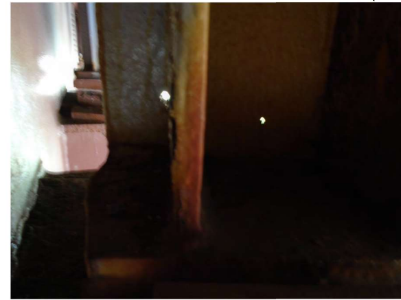
Picture 6: P19 WS SP 20 BM10 NF LOOKING S (R11)
