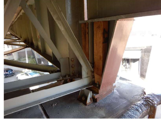
Photo 4: Pier 24, Bolster at Girder G57 with Timber Cribbing (Looking North)
