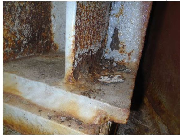
Picture 14: P21 BM14 BEAM END SF LOOKING NW (R20)
