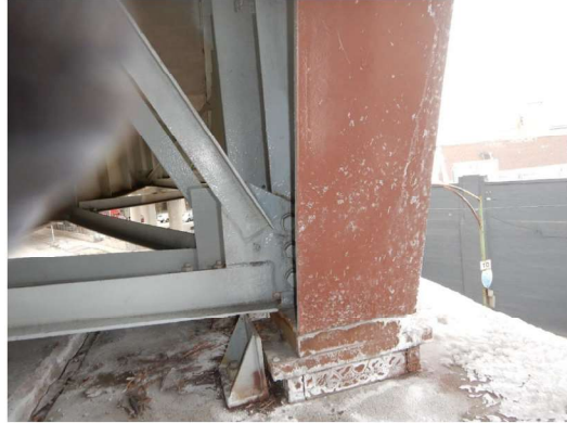
Photo 2: Pier 24, Bolster at Girder G57 (Looking Northwest)
