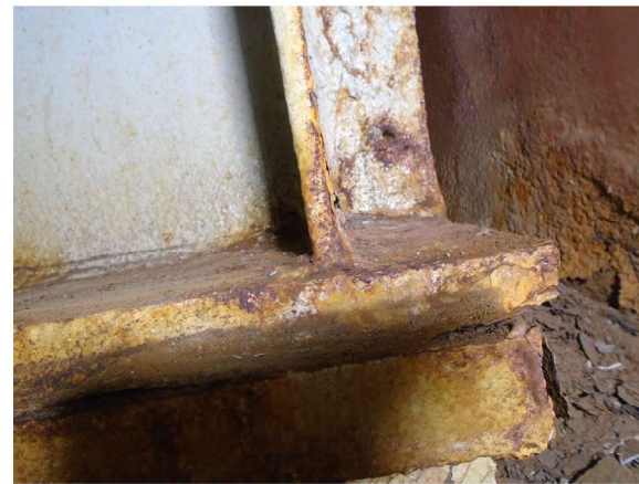
Picture 15: P21 WS SP 22 BM 13 SS LOOKING NE (R21)
