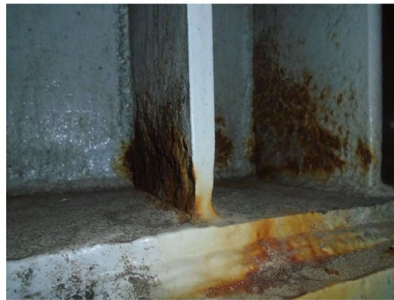
Picture 3: P19 WS SP 20 BM 15 SS LOOKING NE (R9)
