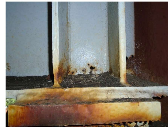
Picture 17: P22 BM9 BEAM END S LOOKING N (R25)
