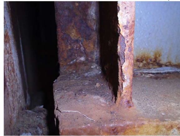
Picture 16: P21 WS SP 22 BM 12 NS LOOKING S (R22)
