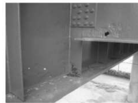
Photo 7: Span C15, Pier C15, G5-C
