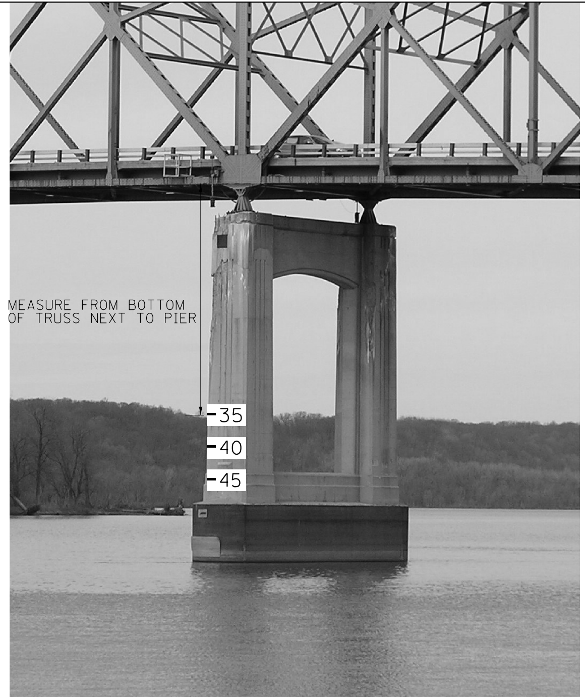
PIER 6 LOOKING UPSTREAM
