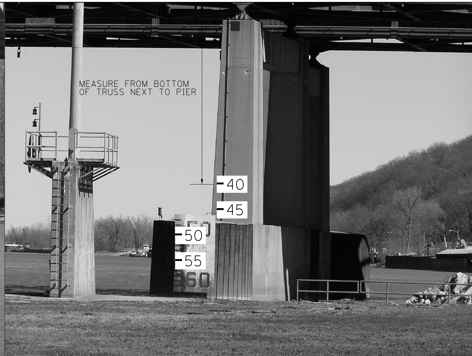
PIER 10 LOOKING UPSTREAM
