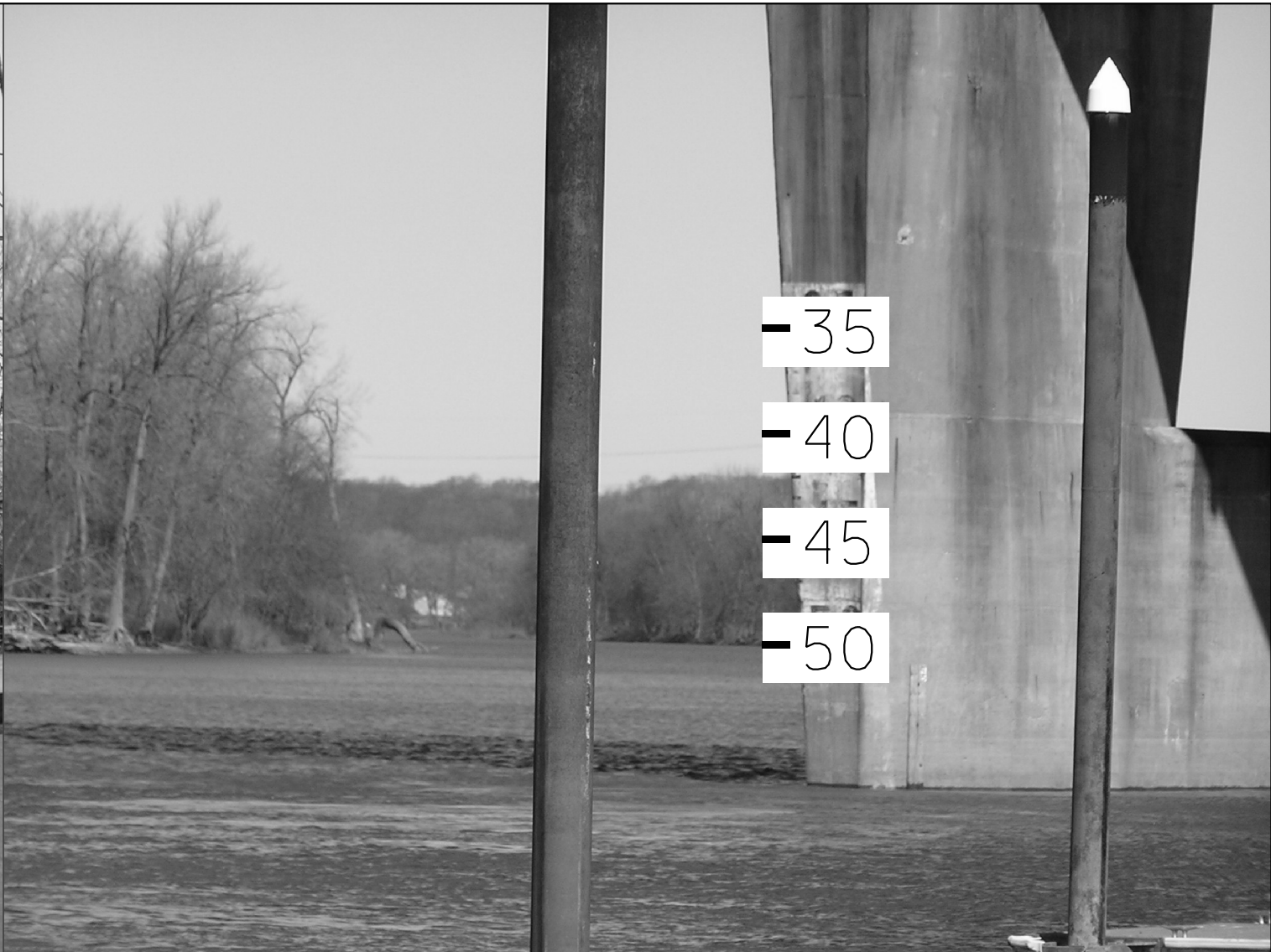
PIER 8 LOOKING UPSTREAM
