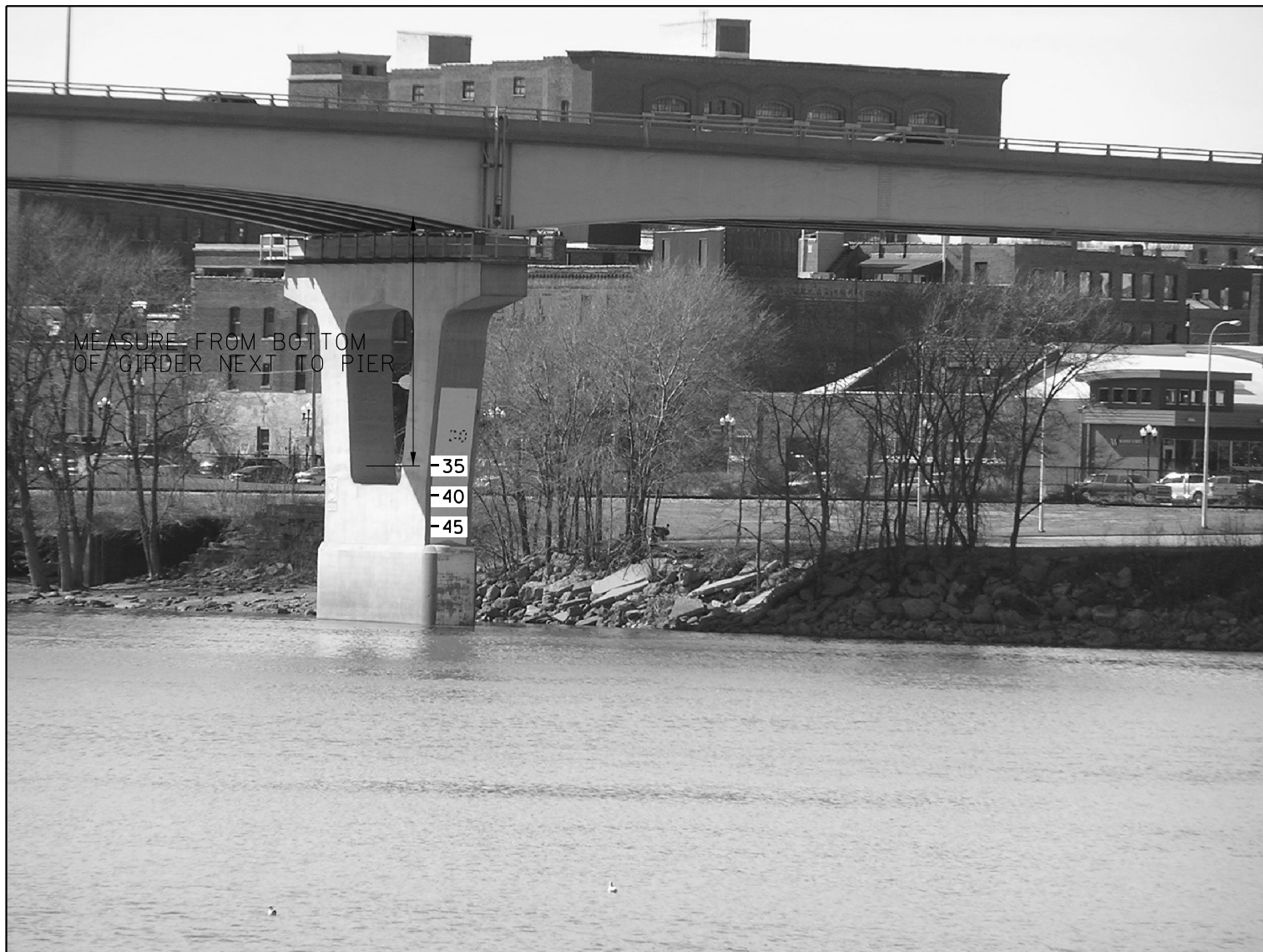
PIER 7 LOOKING DOWNSTREAM
