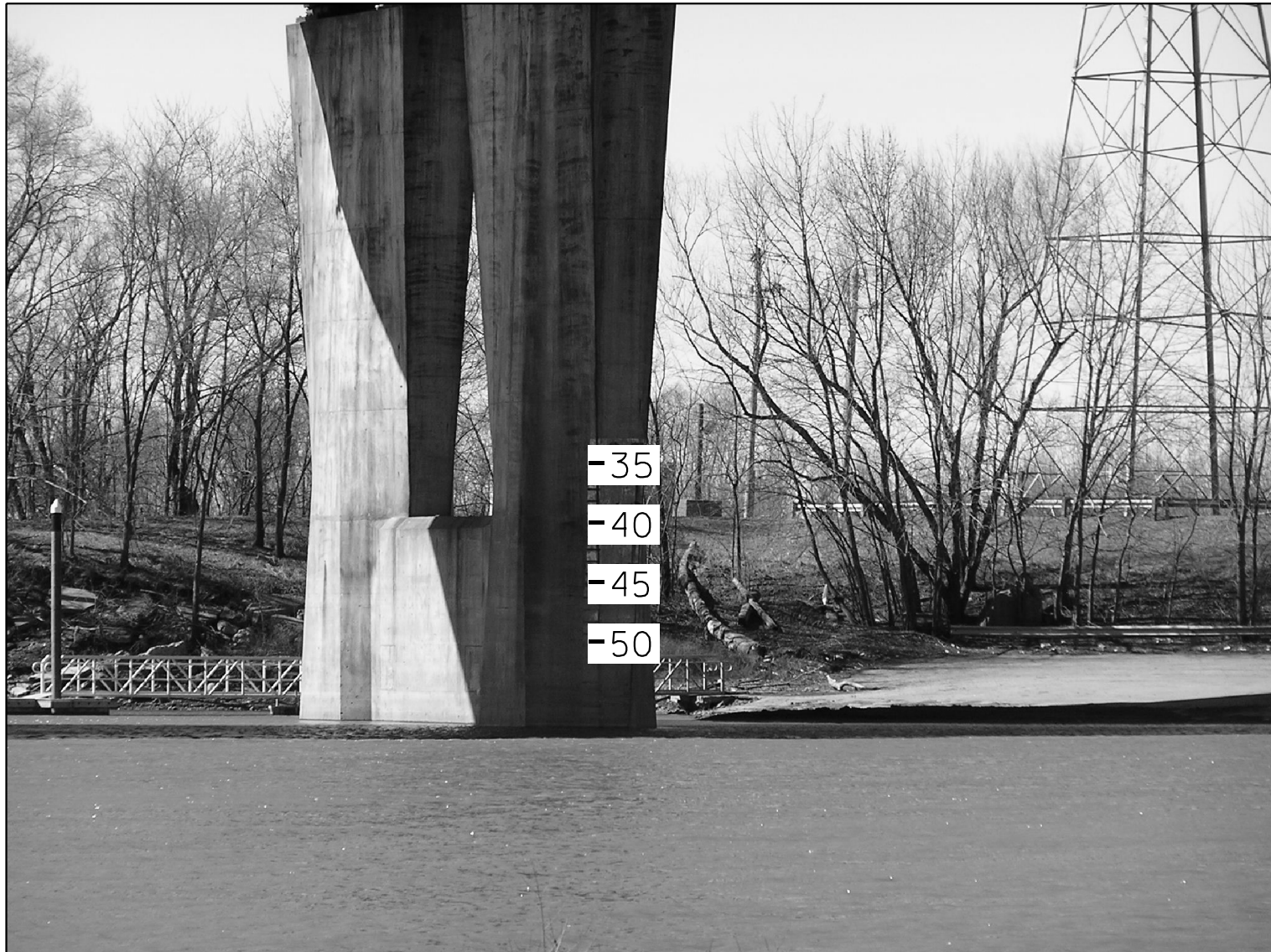
PIER 7 LOOKING DOWNSTREAM
