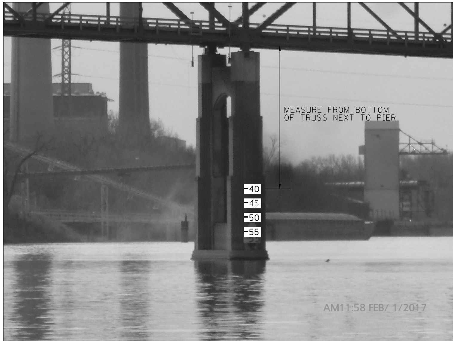
PIER 6 LOOKING DOWNSTREAM
