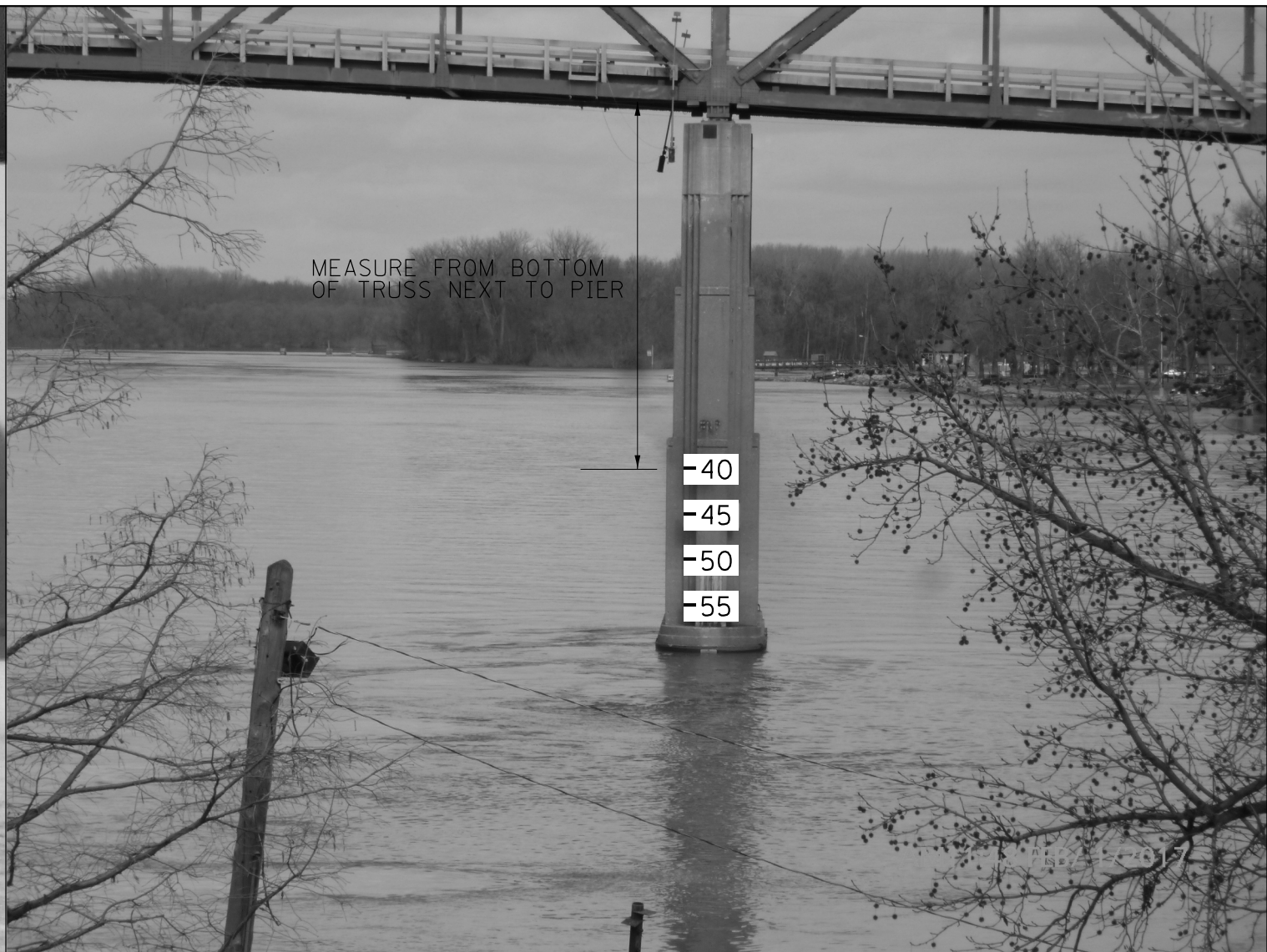
PIER 7 LOOKING UPSTREAM
