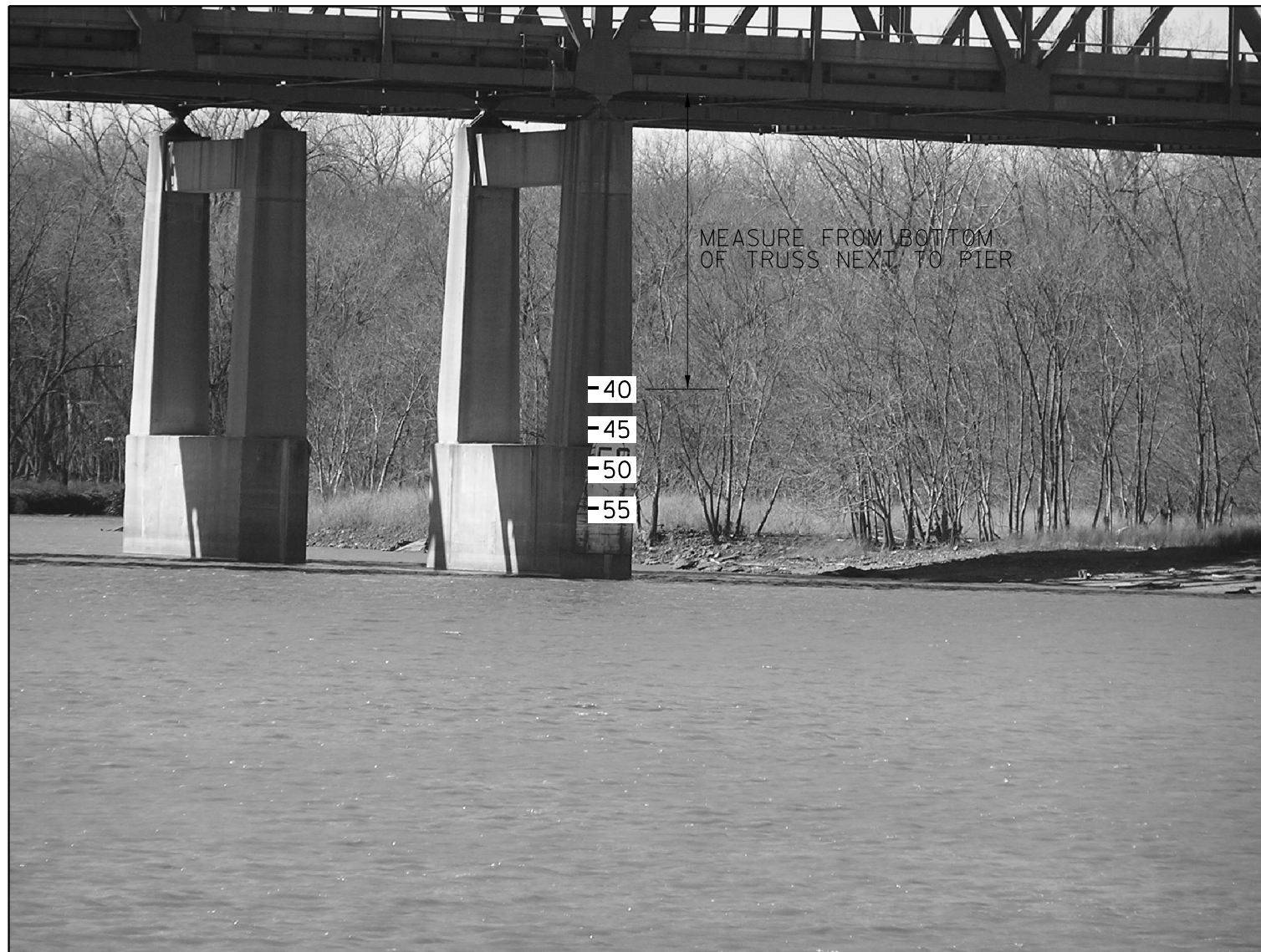
PIER 9 LOOKING DOWNSTREAM
