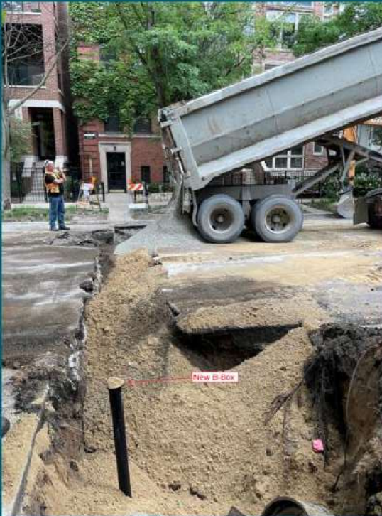
Backfill with sand and pea gravel
