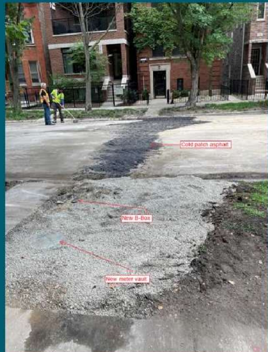
Cold patch asphalt on road
