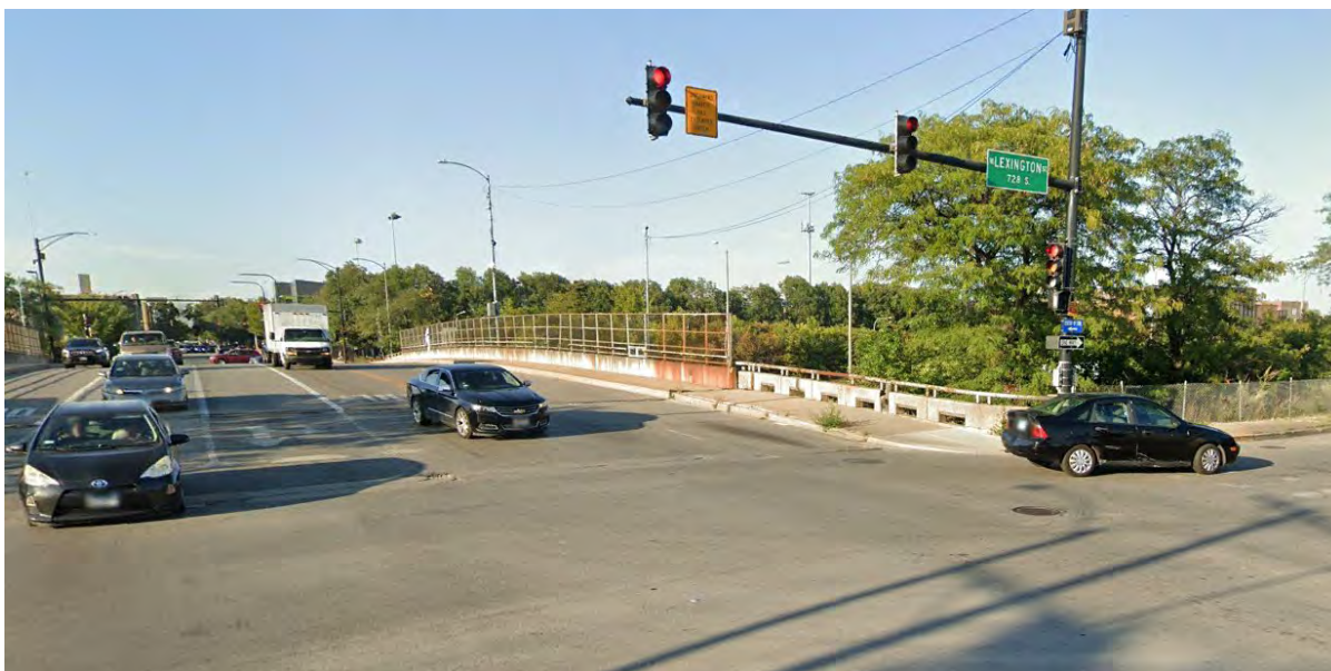
Exhibit 2a – Existing Laramie Avenue Bridge, Looking North along Laramie Avenue
