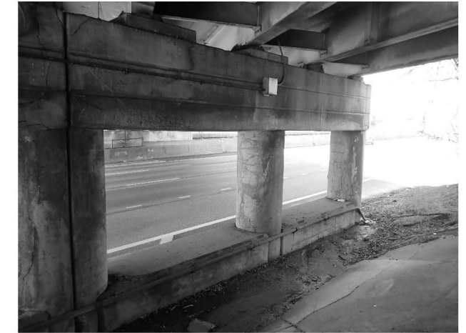
CONDUIT ON PIER 1 (Looking Northwest)
