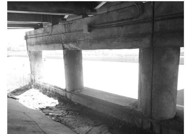
CONDUIT ON PIER 1 (Looking Southwest)
