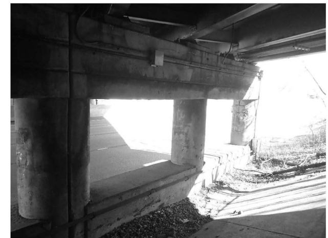
CONDUIT ON PIER 3 (Looking Southeast)
