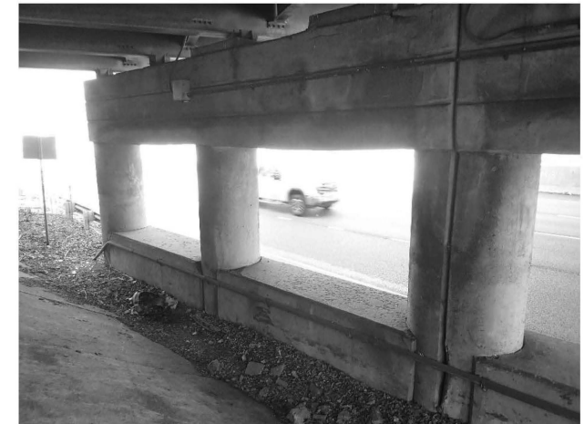
CONDUIT ON PIER 3 (Looking Northeast)
