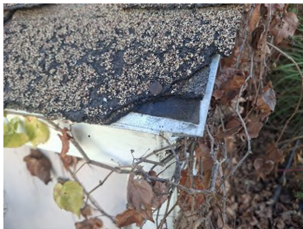
HA-29: Brown Asphalt Shingles HA-30: Black Tar Paper under HA-29
