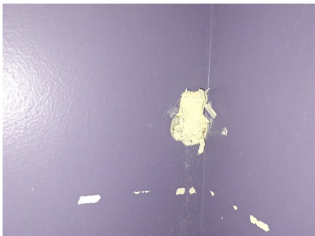
HA-9: White Gypsum Board (painted purple) HA-11: White Joint Compound associated with HA-9 HA-12: Beige Drywall Tape associated with HA-9
