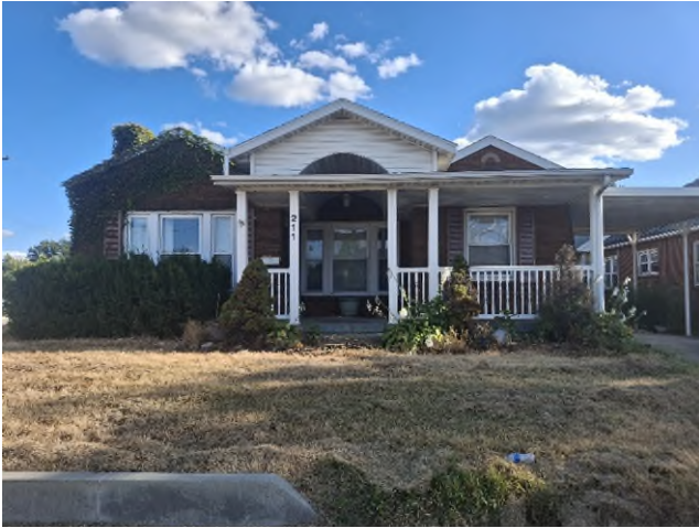
Exterior of Building – Front
