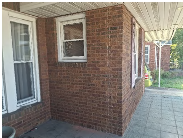
HA-18: Red Brick HA-19: Red Mortar associated with HA-18
