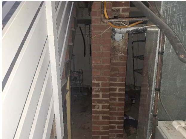
HA-25: Red Brick of Flue HA-26: Gray Mortar associated with HA-25
