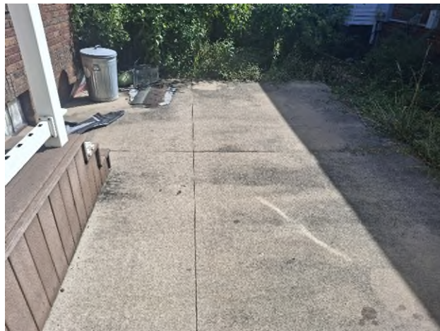
HA-8: Gray Concrete Foundation
