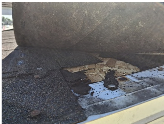
HA-27: Brown Asphalt Shingles HA-28: Black Tar Paper under HA-27
