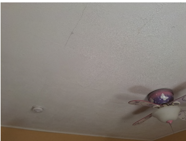
HA-38: White Gypsum Board Ceiling
