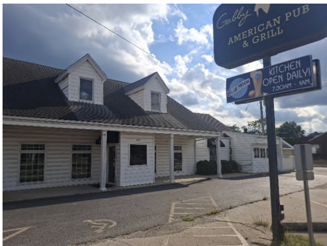
Exterior of Building – Front
