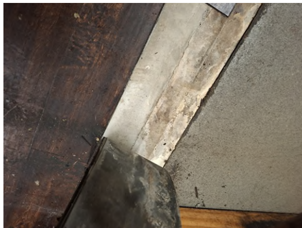
HA-20: Brown Vinyl Flooring HA-21: Beige Mastic associated with HA-20
