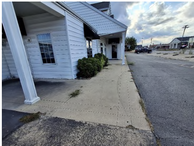
HA-9: Gray Concrete Foundation
