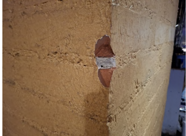
HA-32: Red Brick of Flue HA-33: Gray Mortar associated with HA-32
