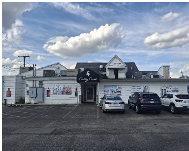
Exterior of Building - Back
