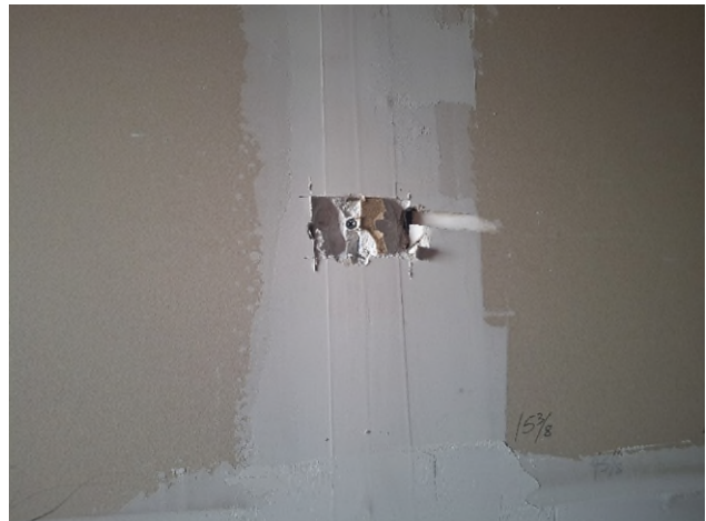
HA-35: White Joint Compound associated with HA-34 HA-36: Beige Drywall Tape associated with HA-34
