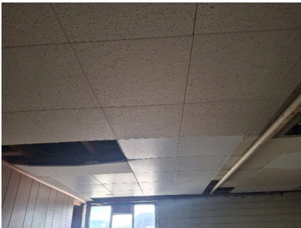
HA-3: Tan 12" x 12" Ceiling Tile (pinhole) HA-4: White 12" x 12" Ceiling Tile
