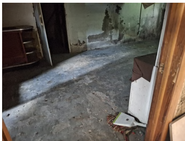
HA-25: Gray Concrete Foundation
