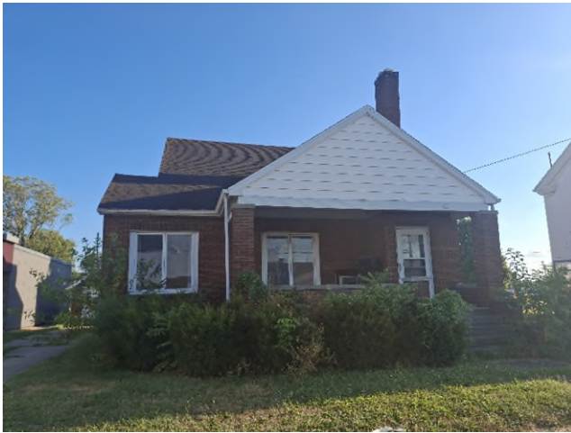
Exterior of Building – Front
