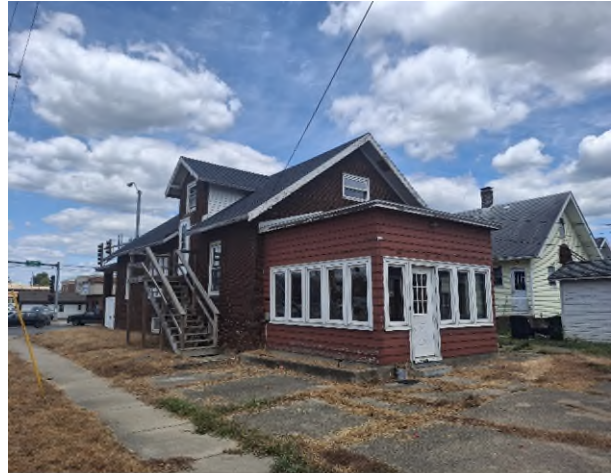
Exterior of the Building - Back
