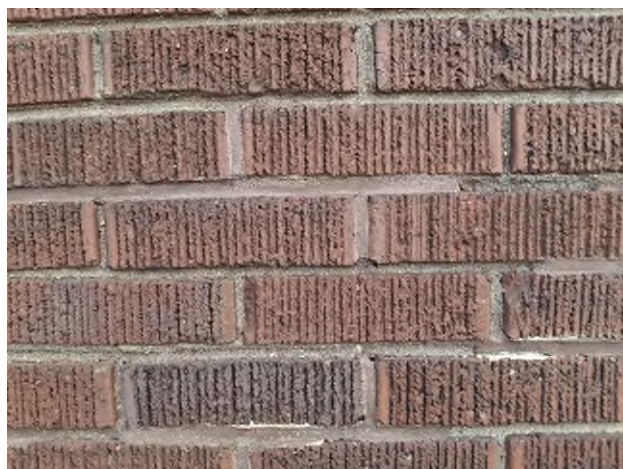
HA-16: Red Brick HA-17: Red Mortar associated with HA-16
