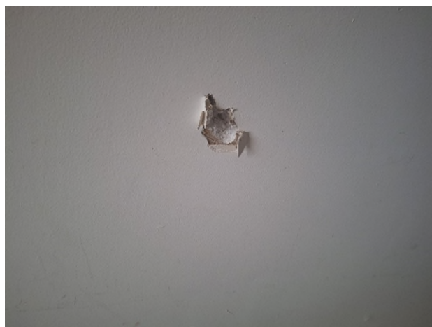
HA-11: Beige Drywall Tape associated with HA-10 HA-12: White Joint Compound associated with HA-10
