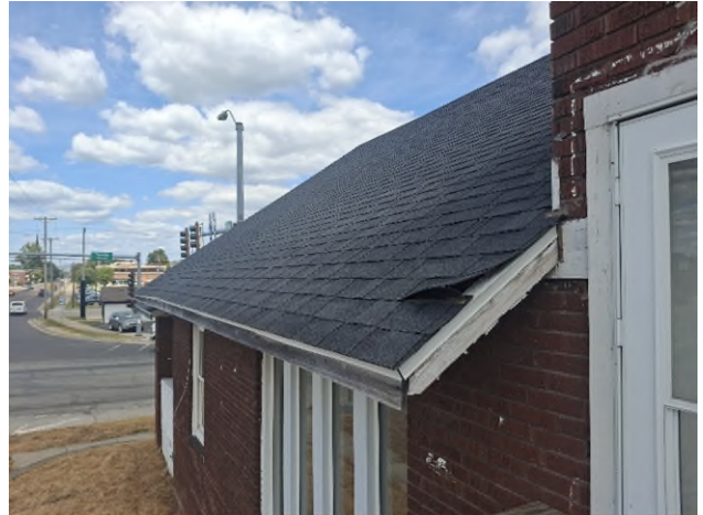
HA-22: Black Asphalt Roof Shingles
