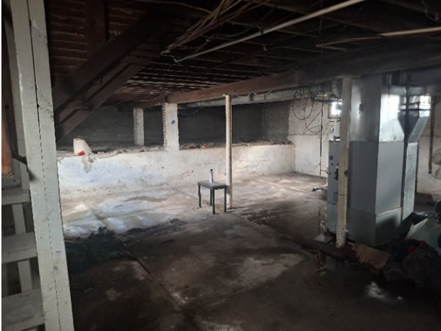
HA-27: Gray Concrete Foundation
