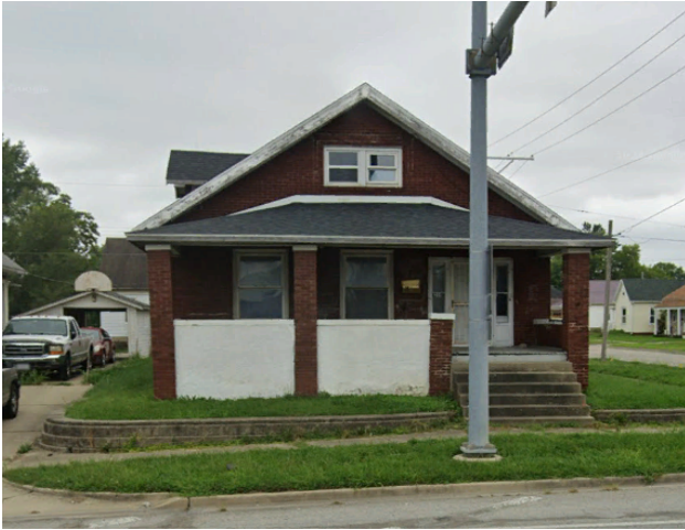
Exterior of Building – Front
