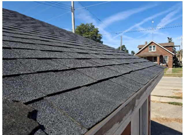
HA-24: Black Asphalt Roof Shingles
