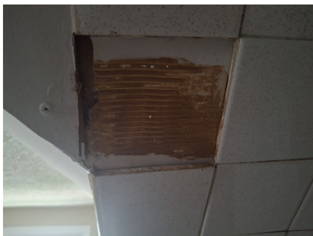
HA-18: White Grout associated with HA-2 HA-19: Beige Adhesive associated with HA-2
