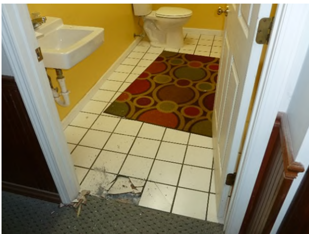
HA-18: White 8" x 8" Ceramic Floor Tile HA-19: Black Tile Grout associated with HA-18 HA-20: Gray Tile Adhesive associated with HA-18 HA-21: Gray Tile Backer Board associated with HA-18
