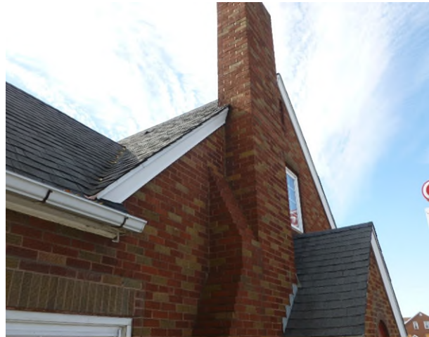
HA-1: Black Asphalt Shingle (top layer) HA-2: Red Asphalt Shingle (middle layer) HA-3: Black Tar Paper (bottom layer)
