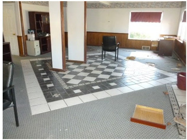
HA-14: Black 12" x 12" Ceramic Floor Tile HA-15: Black Tile Grout associated with HA-14 HA-16: Gray Tile Adhesive associated with HA-14 HA-17: Gray Tile Backer Board associated with HA-14
