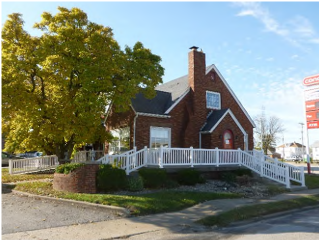
Exterior of Building – Front
