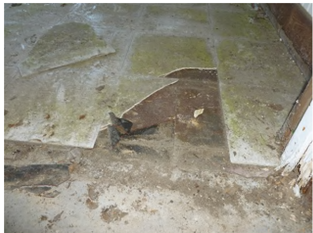
HA-16: Red 9" x 9" Floor Tile HA-17: Black Mastic associated with HA-16
