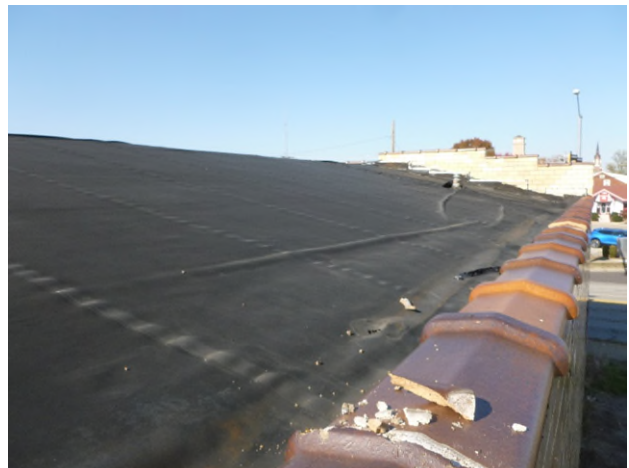
HA-21: Black Roofing Material HA-22: Black Roof Flashing Mastic
