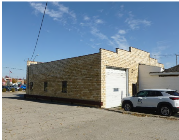
HA-3: Tan Exterior Glazed Block HA-4: Gray Mortar associated with HA-3
