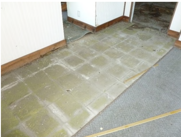
HA-13: Gray 12" x 12" Floor Tile (top layer) HA-14: Gray 12" x 12" Floor Tile (second layer) HA-15: Yellow Mastic associated with HA-14
