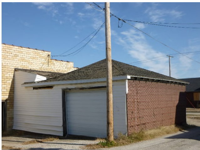
HA-5: Black Asphalt Roof Shingle HA-6: Black Felt Vapor Barrier associated with HA-5
