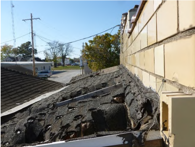
HA-25: Black Roof Flashing Mastic
