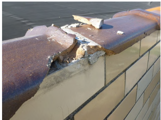
HA-24: Gray Coping Tile Grout
