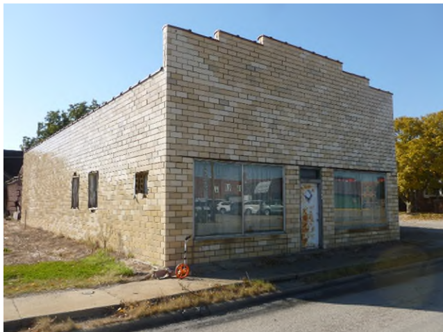
Exterior of Building – Front
