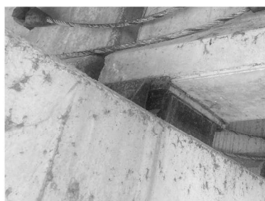
TYPICAL BEARING TO BE CLEANED AND PAINTED
