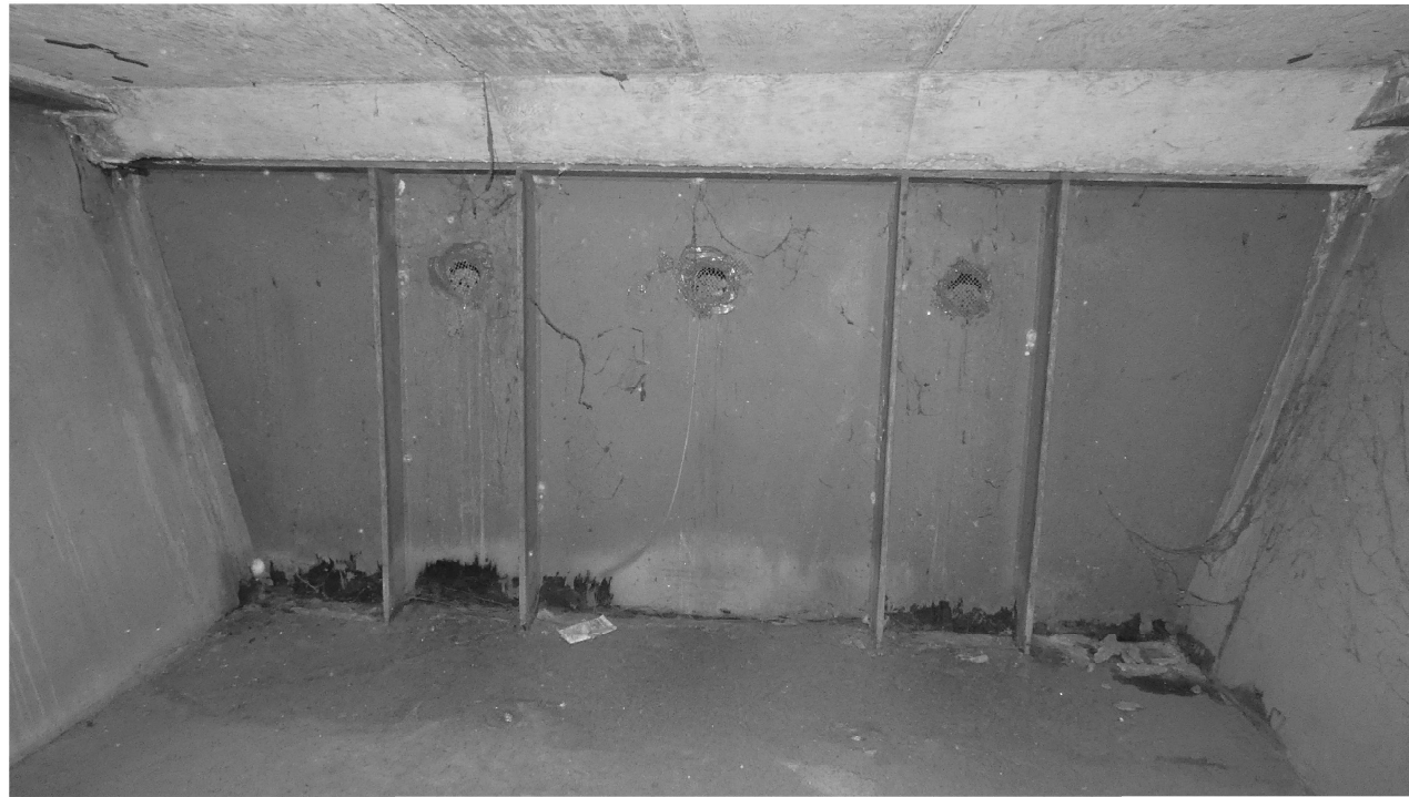
Typical Bulkhead at Abutments
