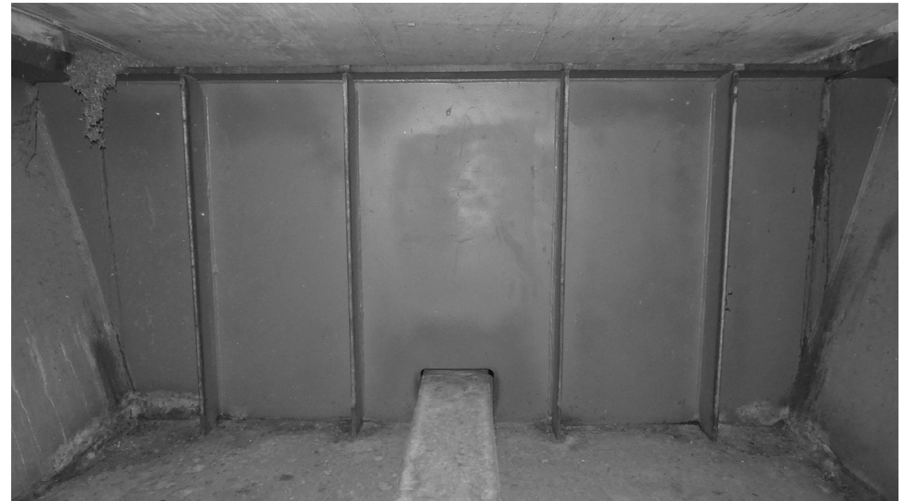
Typical Bulkhead at Pier
