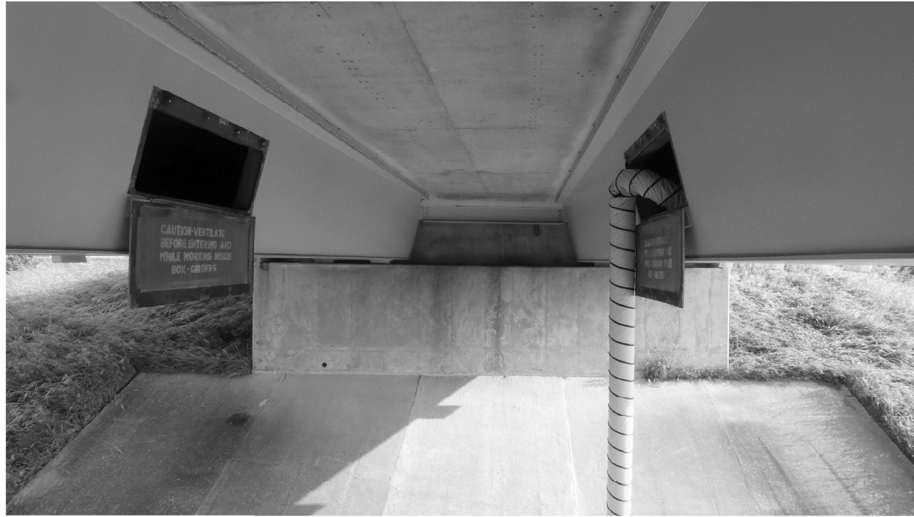
Typical Access Doors for Welded Steel Box-Girders
