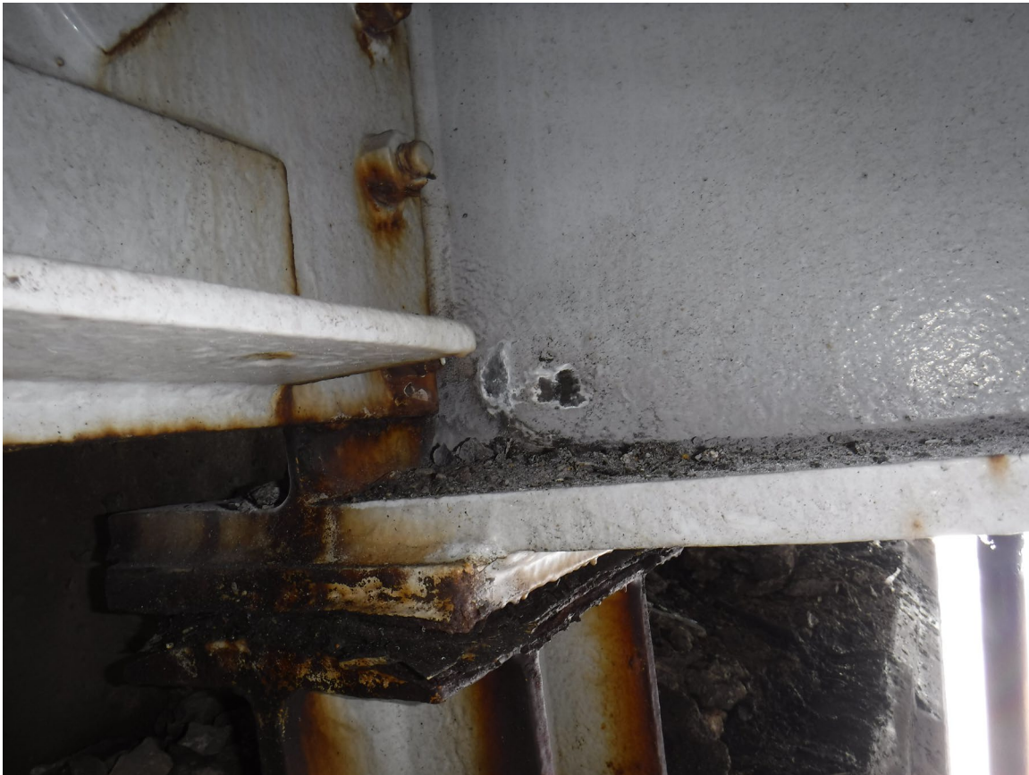
P8; Beam 8; Span 8 Side - Picture 1: West face looking NE
