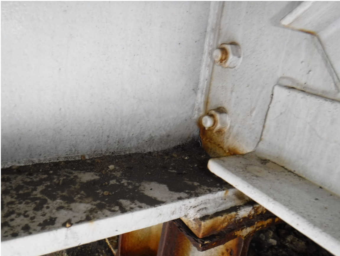
P8; Beam 8; Span 8 side - Picture 3: East face looking NW
