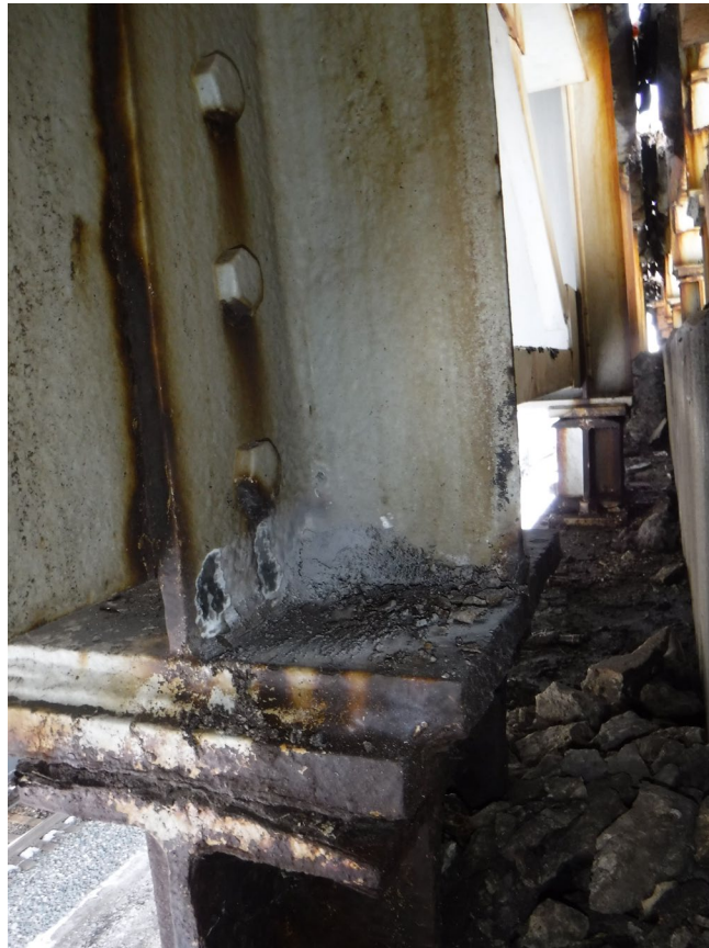
P8; Beam 8; Span 8 side - Picture 4: East face looking SW
