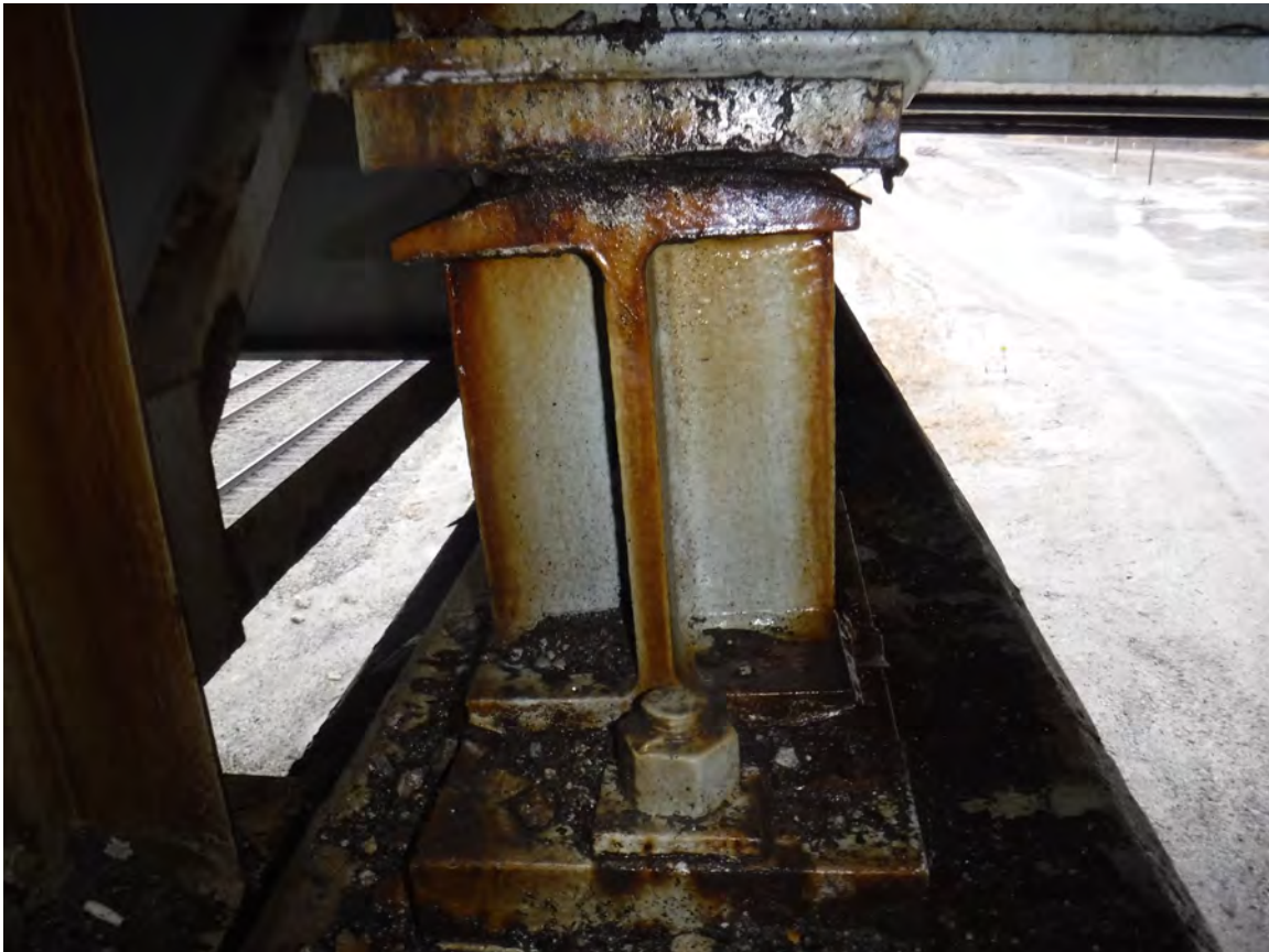
Picture 12: P8; Span 9; Bearing 6; Looking W
