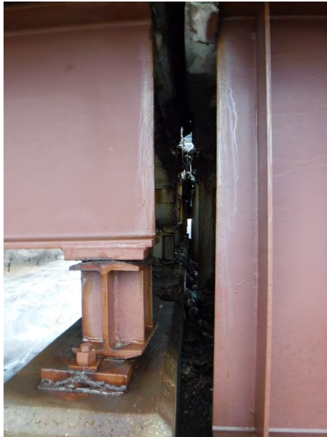
Picture 6: P8, span 9; bearing 1; looking E
