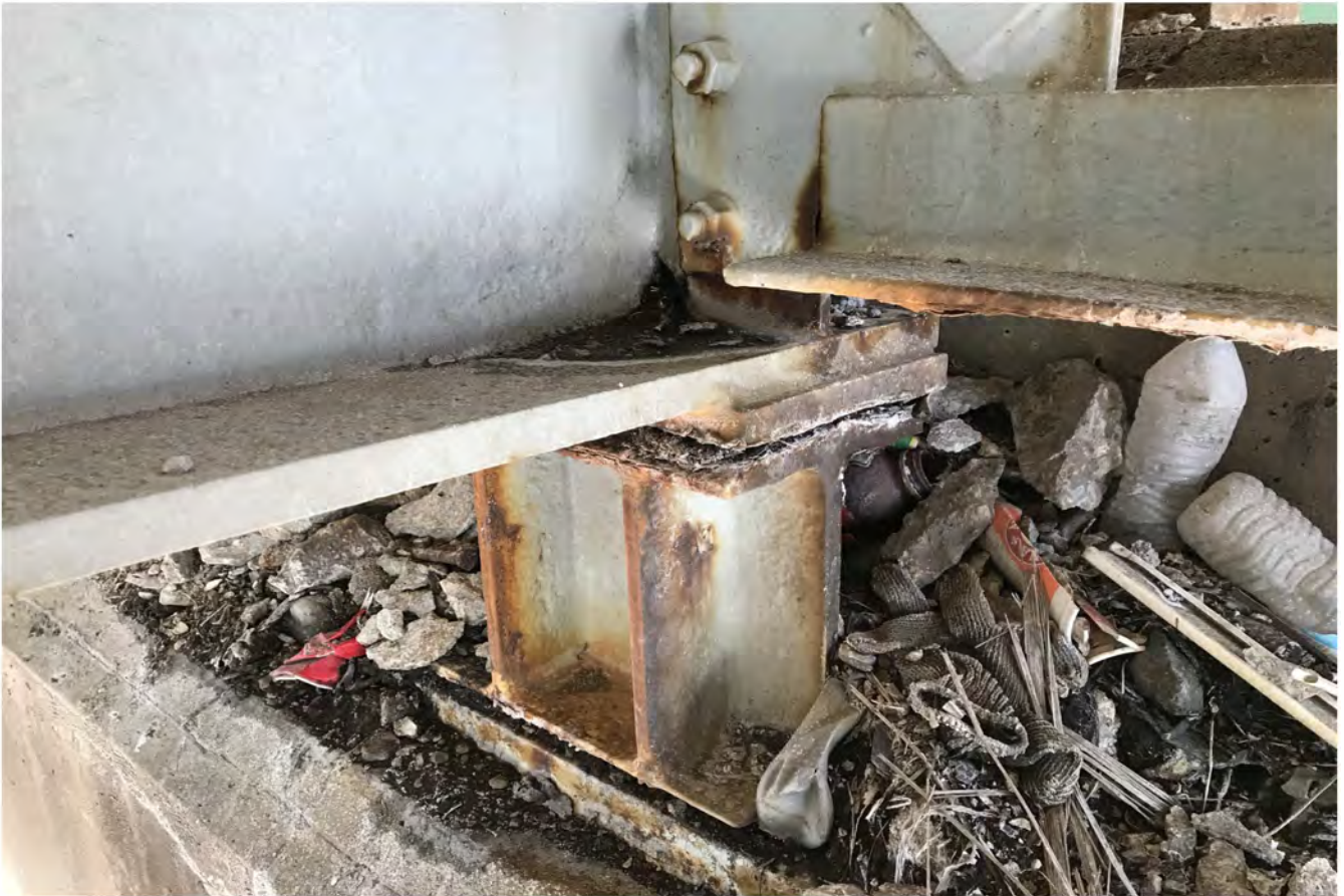
BEAM 9- E FACE-PIER 8S
