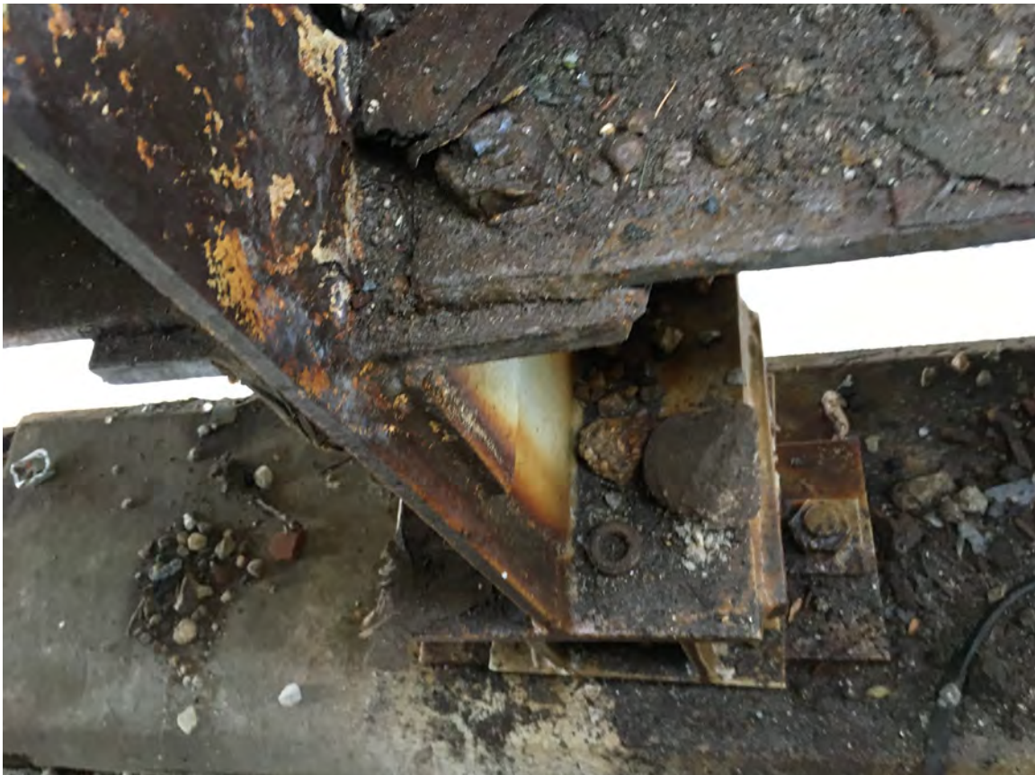
Picture 2: P8; Span 9; Beam 2 end
