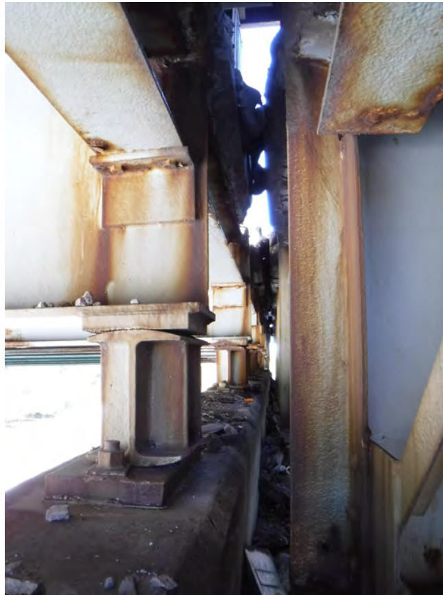
Picture 3: P8; Span 9; Beam 2 end west face.
