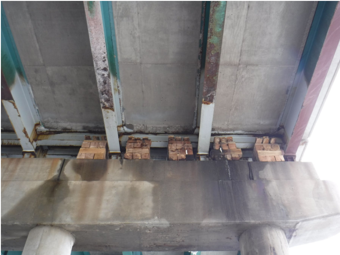
Picture 20: Pier 8 West End; North Face; Looking S
