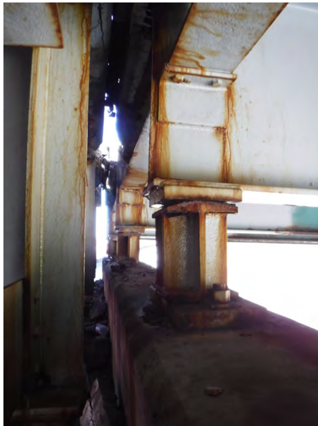
Picture 4: P8; Span 9; Beam 4 end east face
