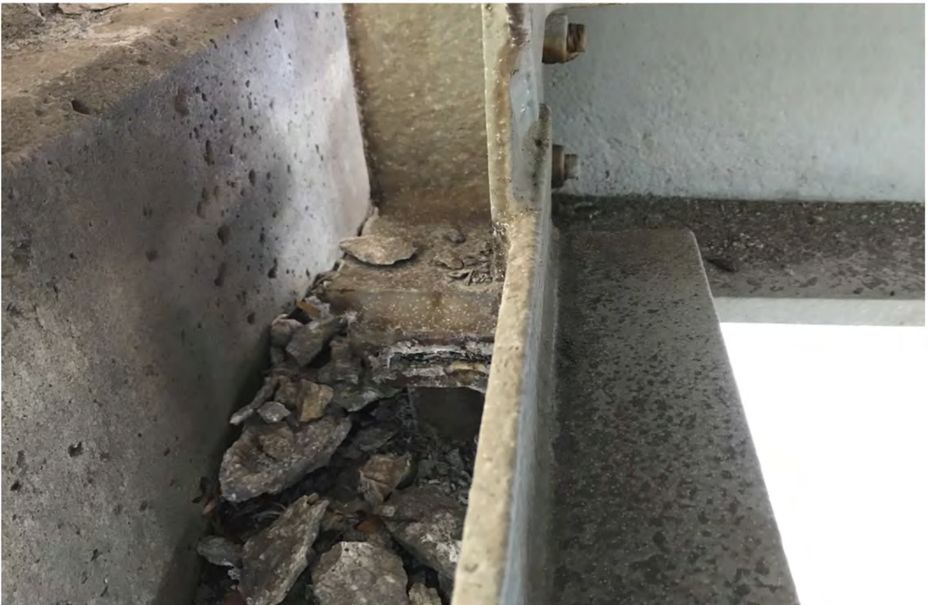
BEAM 9- W FACE- PIER 8S
