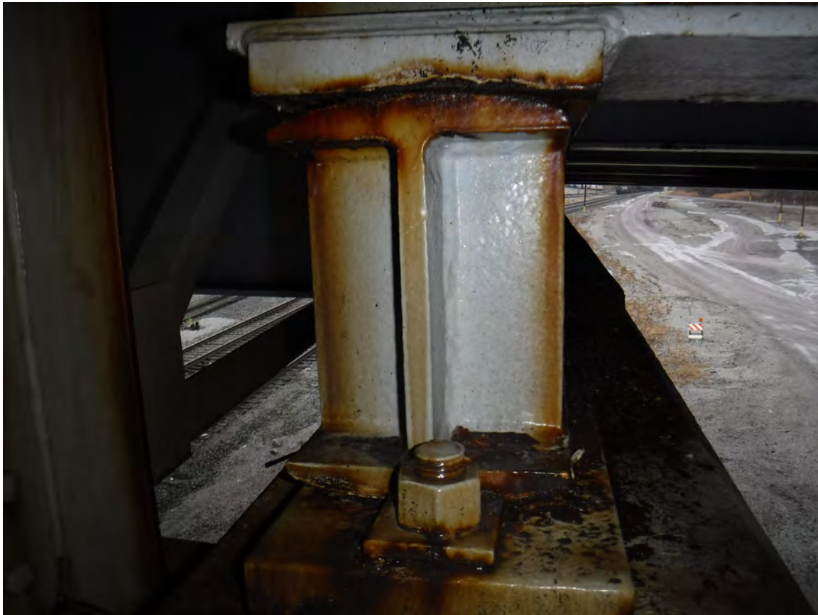
Picture 13: P8; Span 9; Bearing 7; Looking W
