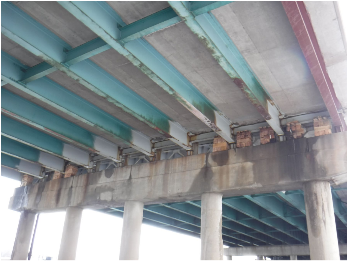
Picture 18: Pier 8; North Face; Looking SE
