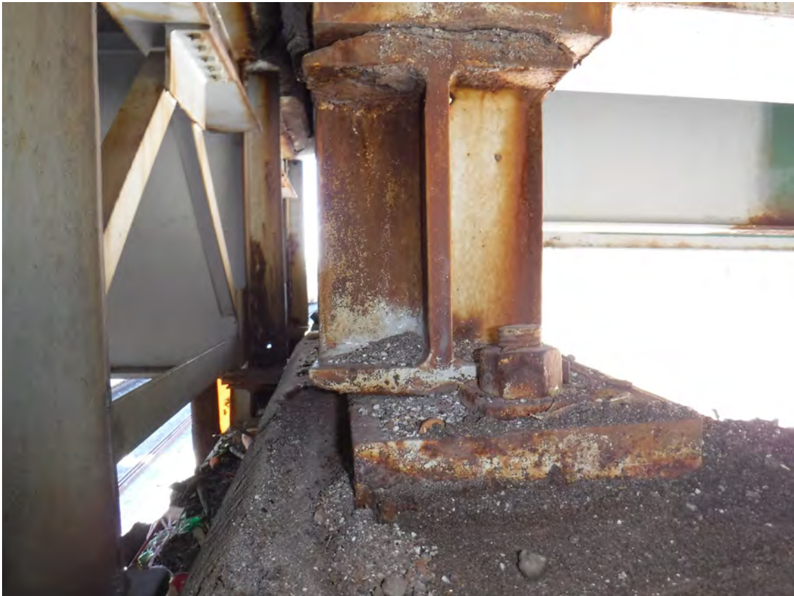
Picture 5: P8; Span 9; Beam 3 bearing; looking west
