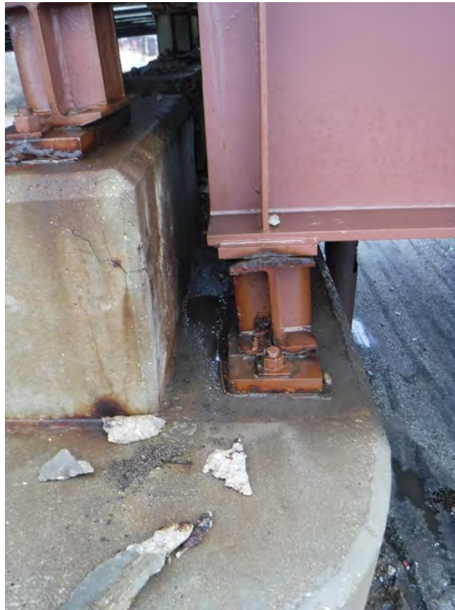
Picture 7: P8; Span 9; Looking E
