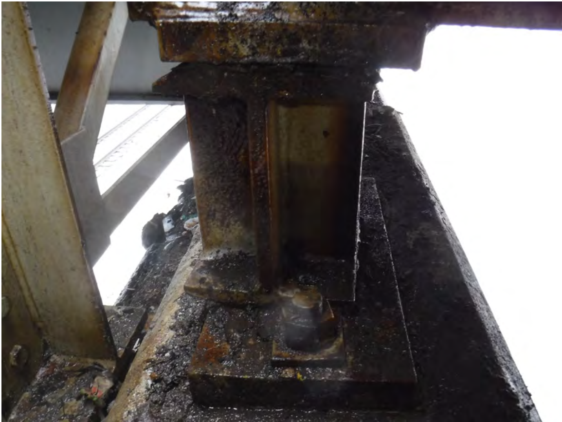
Picture 9: P8; Span 9; Bearing 3; Looking W
