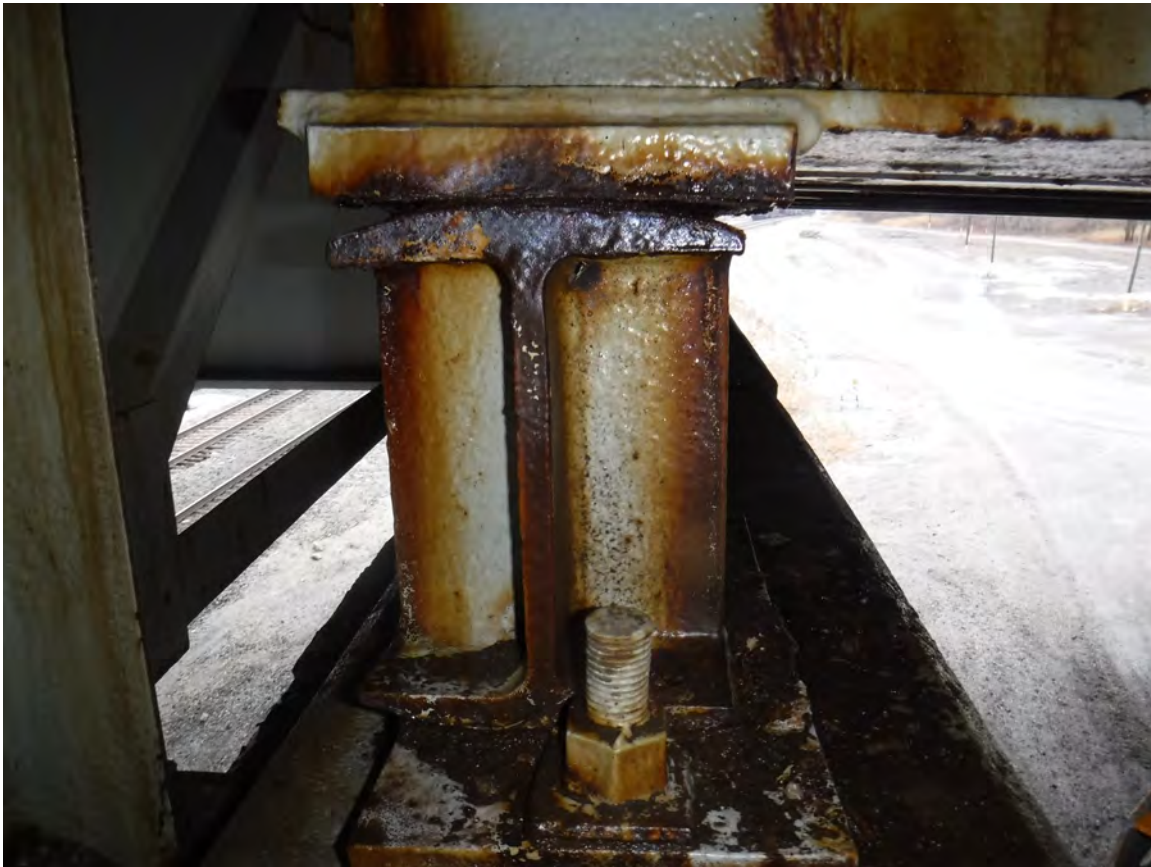
Picture 15: P8; Span 9; Bearing 8; Looking W
