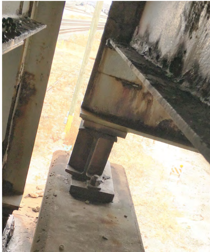
Picture 1: P8; Span 9; Beam 1 Looking W.
