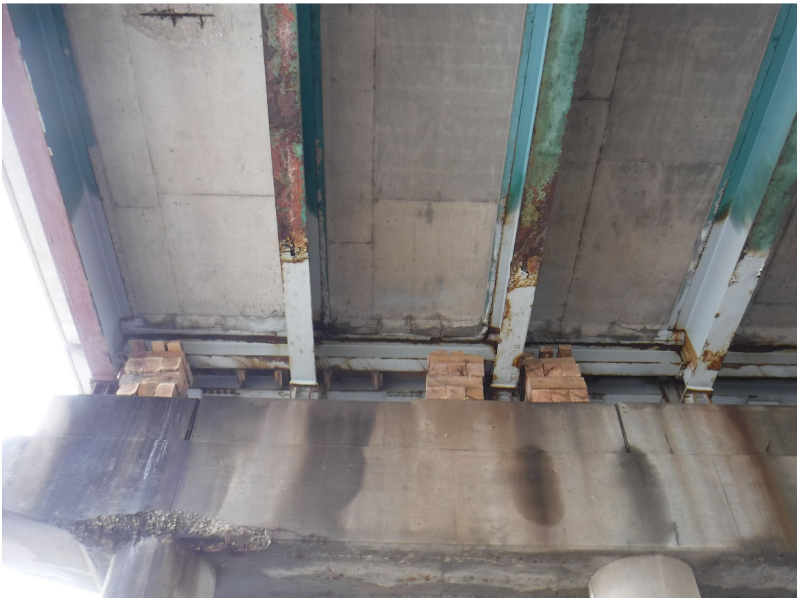
Picture 21: Pier 8 East End; North Face; Looking S
