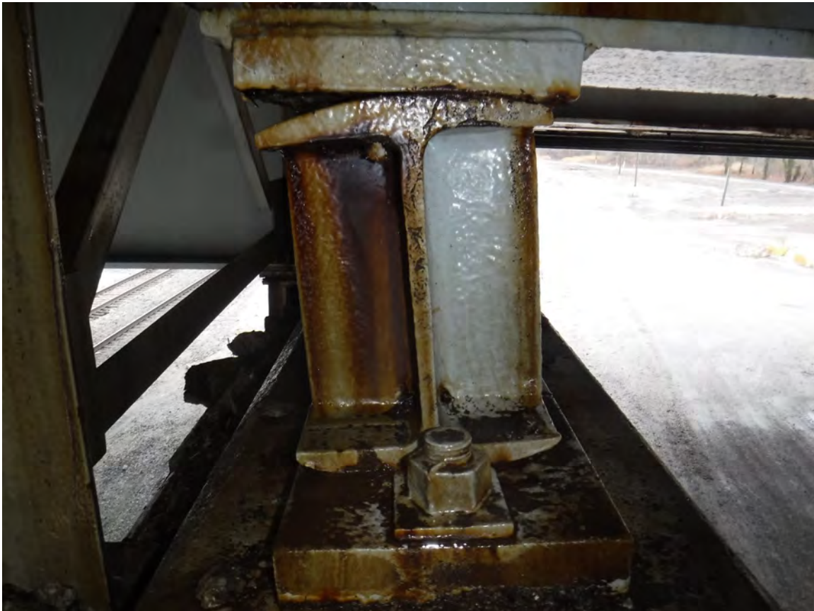
Picture 16: P8; Span 9; Bearing 9; Looking W
