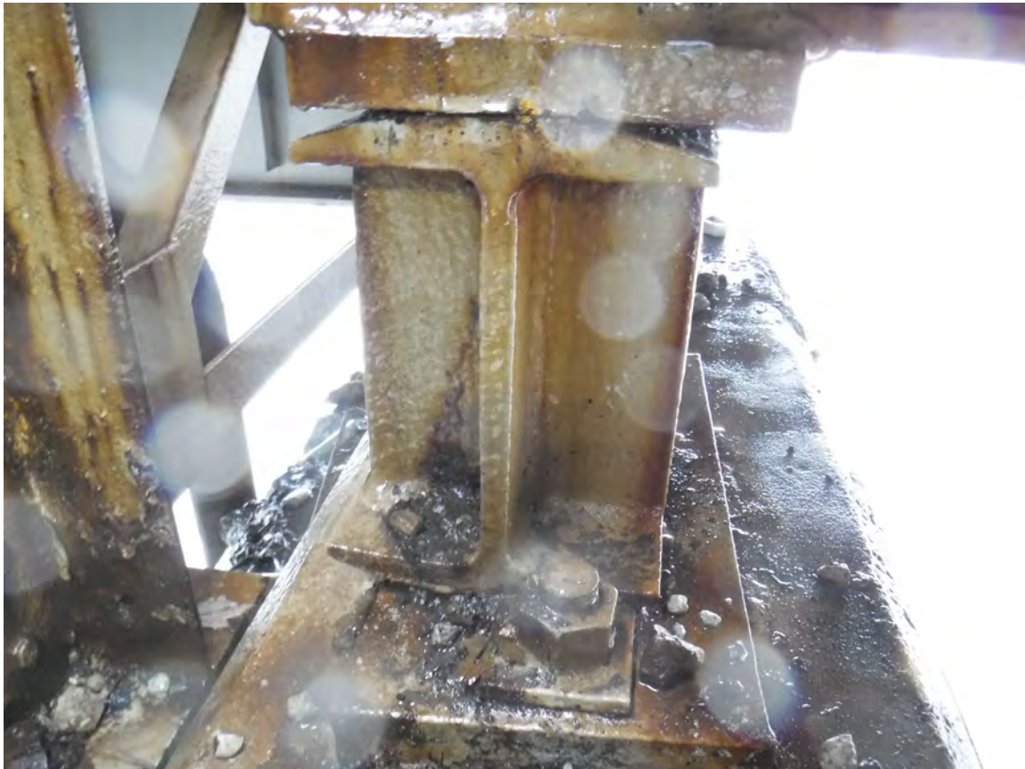
Picture 8: P8; Span 9; Bearing 2; Looking W
