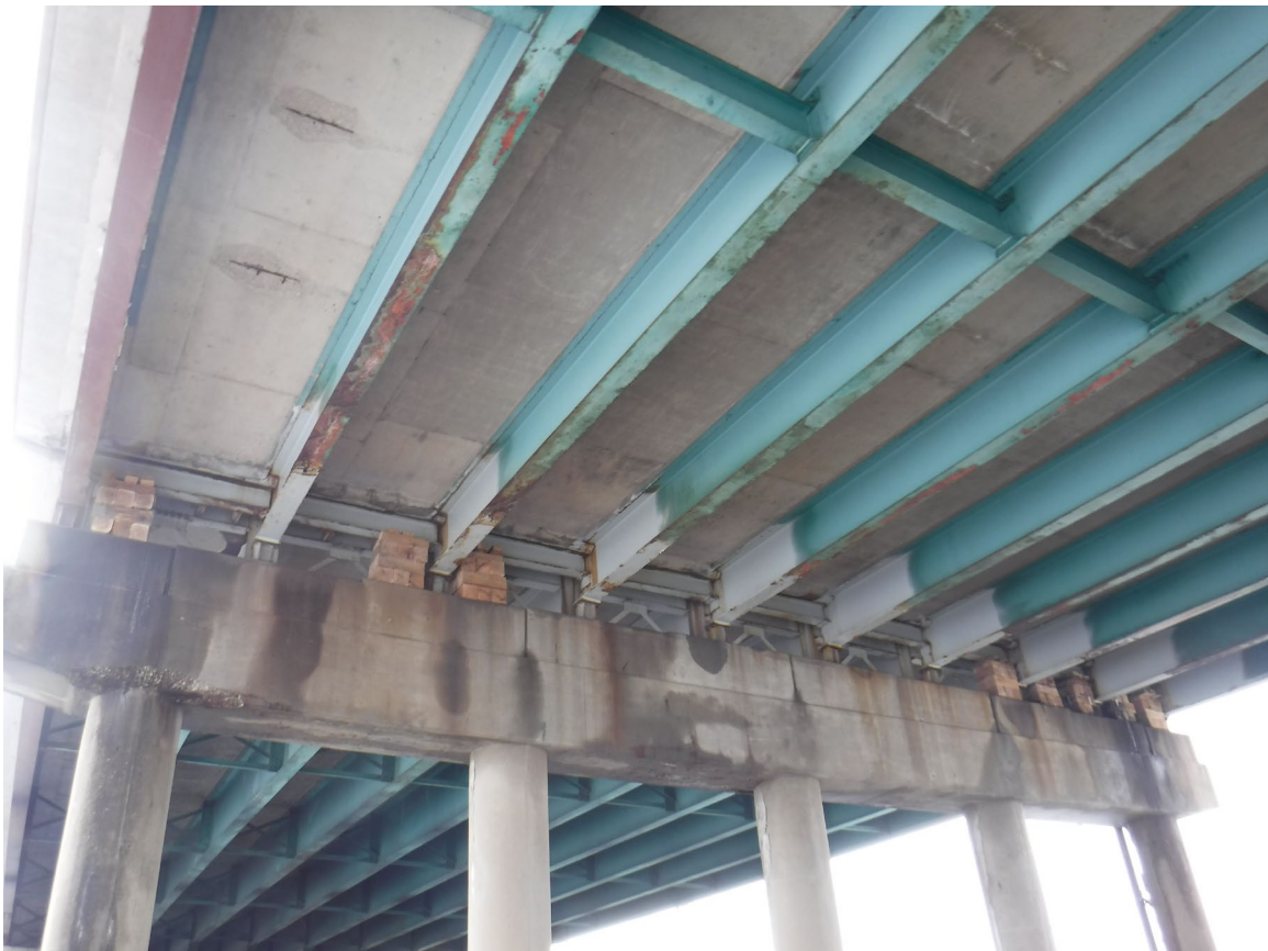
Picture 19: Pier 8; North Face; Looking SW
