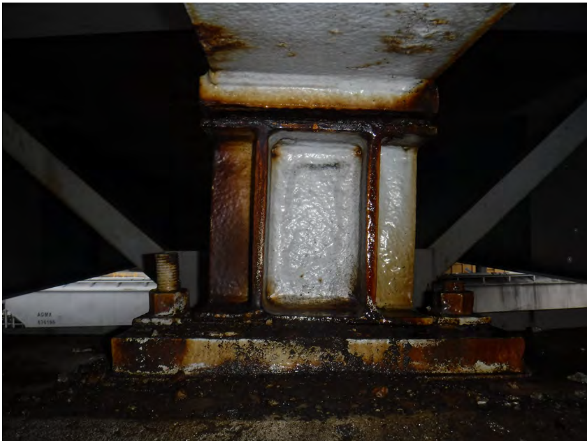
Picture 14: P8; Span 9; Bearing 8; Looking S
