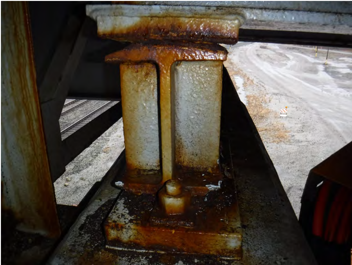
Picture 11: P8; Span 9; Bearing 5; Looking W
