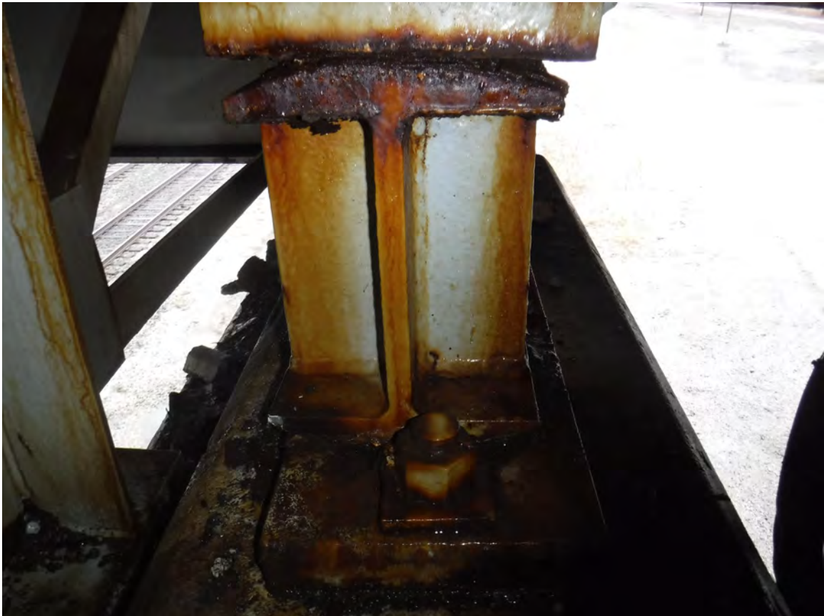
Picture 10: P8; Span 9; Bearing 4; Looking W
