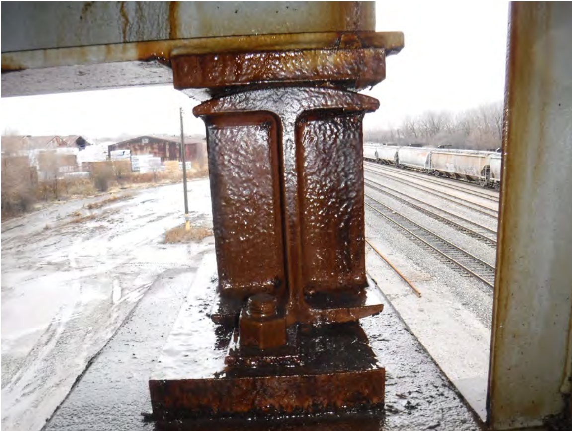
Picture 17: P8; Span 9; Bearing 10; Looking E
