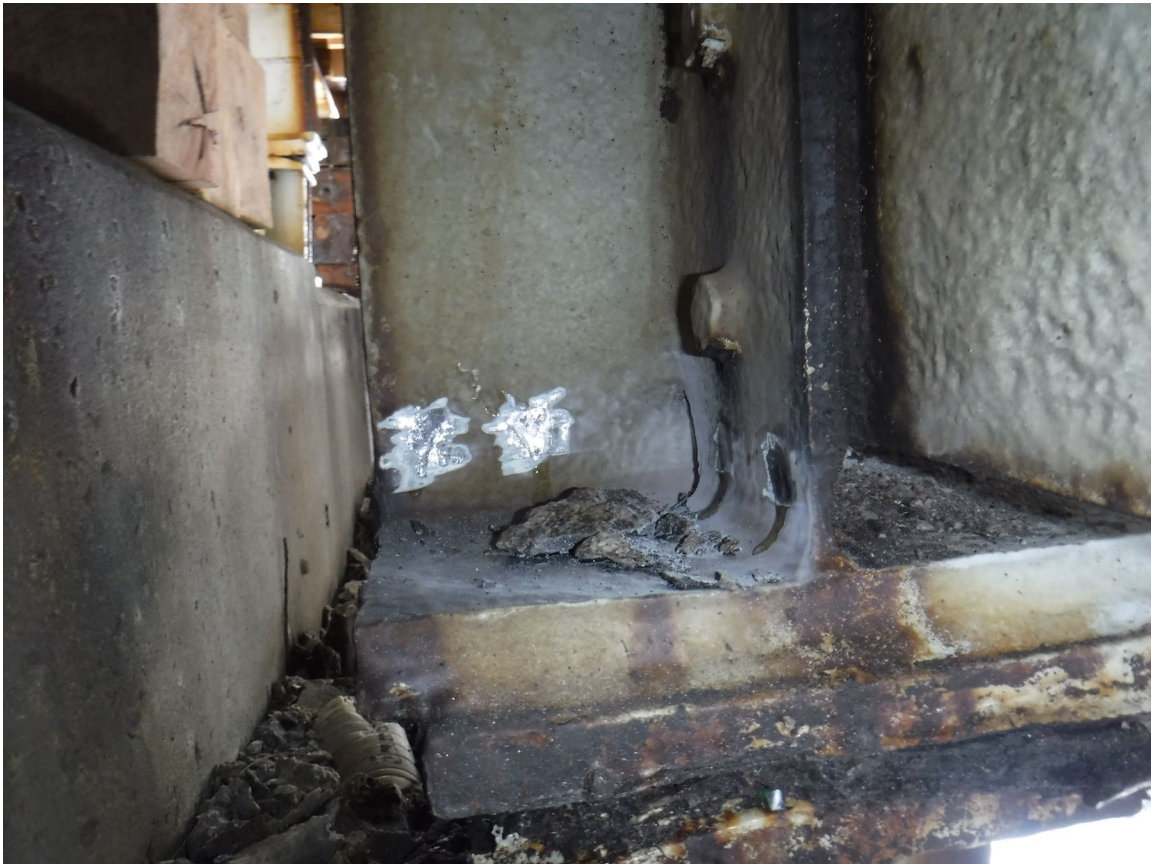
P8; Beam 8; Span 8 side - Picture 2: West face Looking SE
