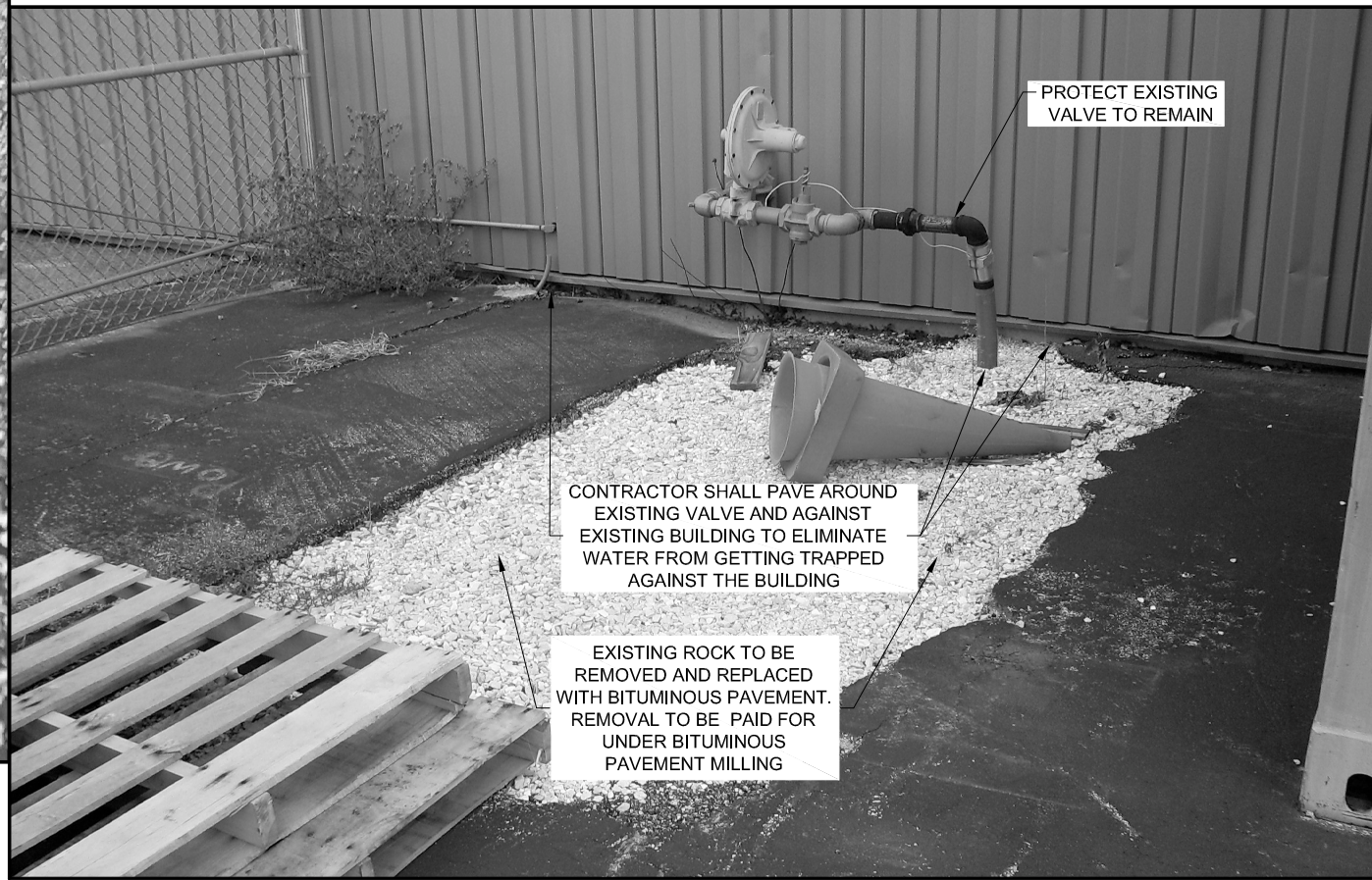
PHOTO 3 - IDA HANGAR (NORTH SIDE)
