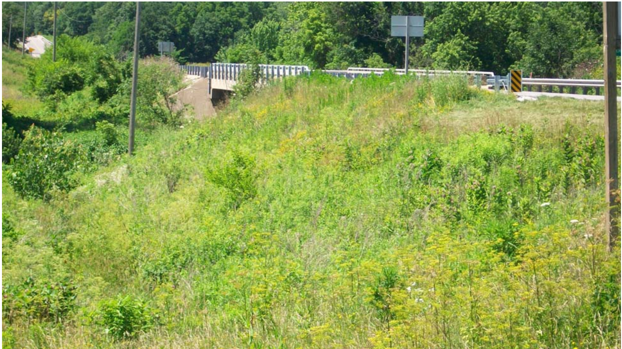
Photo 2 South East Ditch
