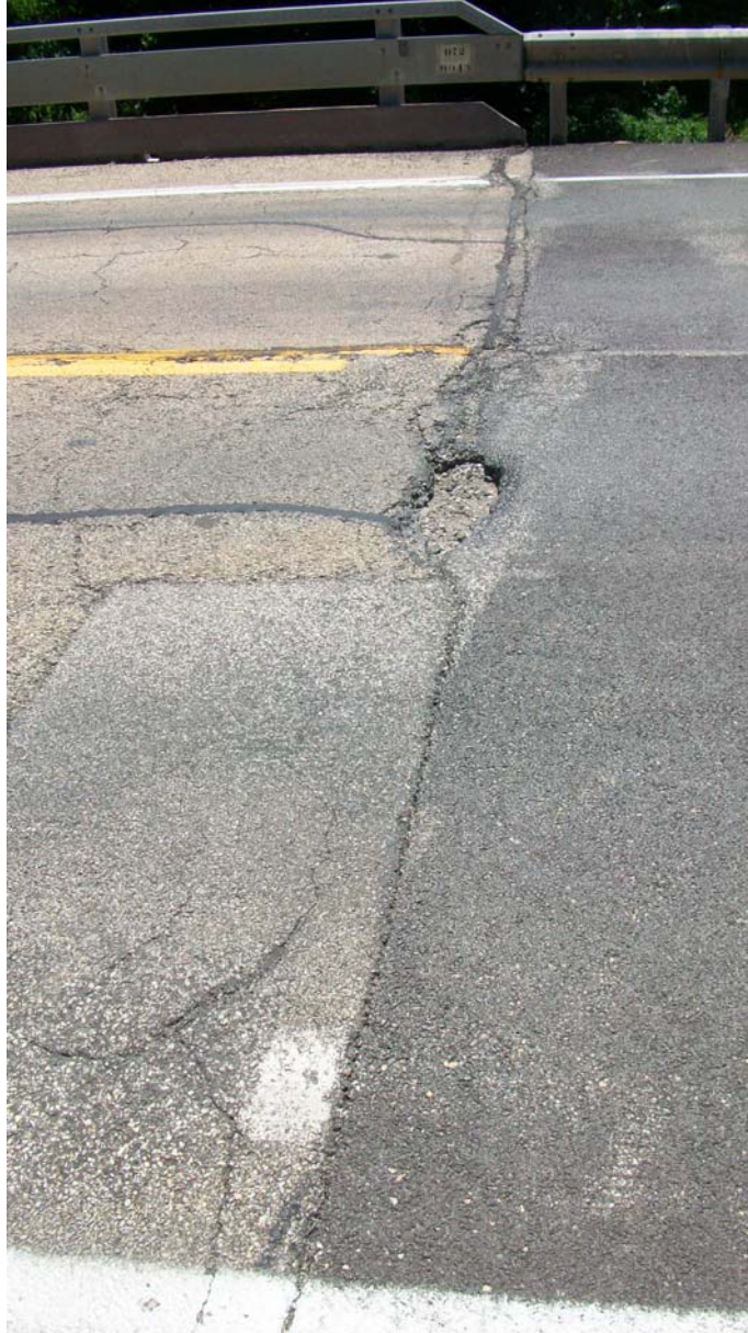
Photo 13 West Bridge Joint
