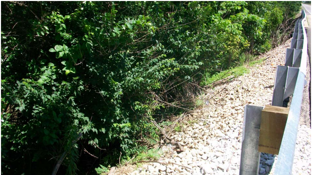
Photo 4 North West Ditch
