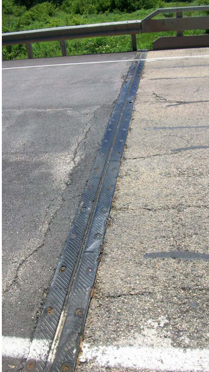
Photo 11 East Bridge Joint
