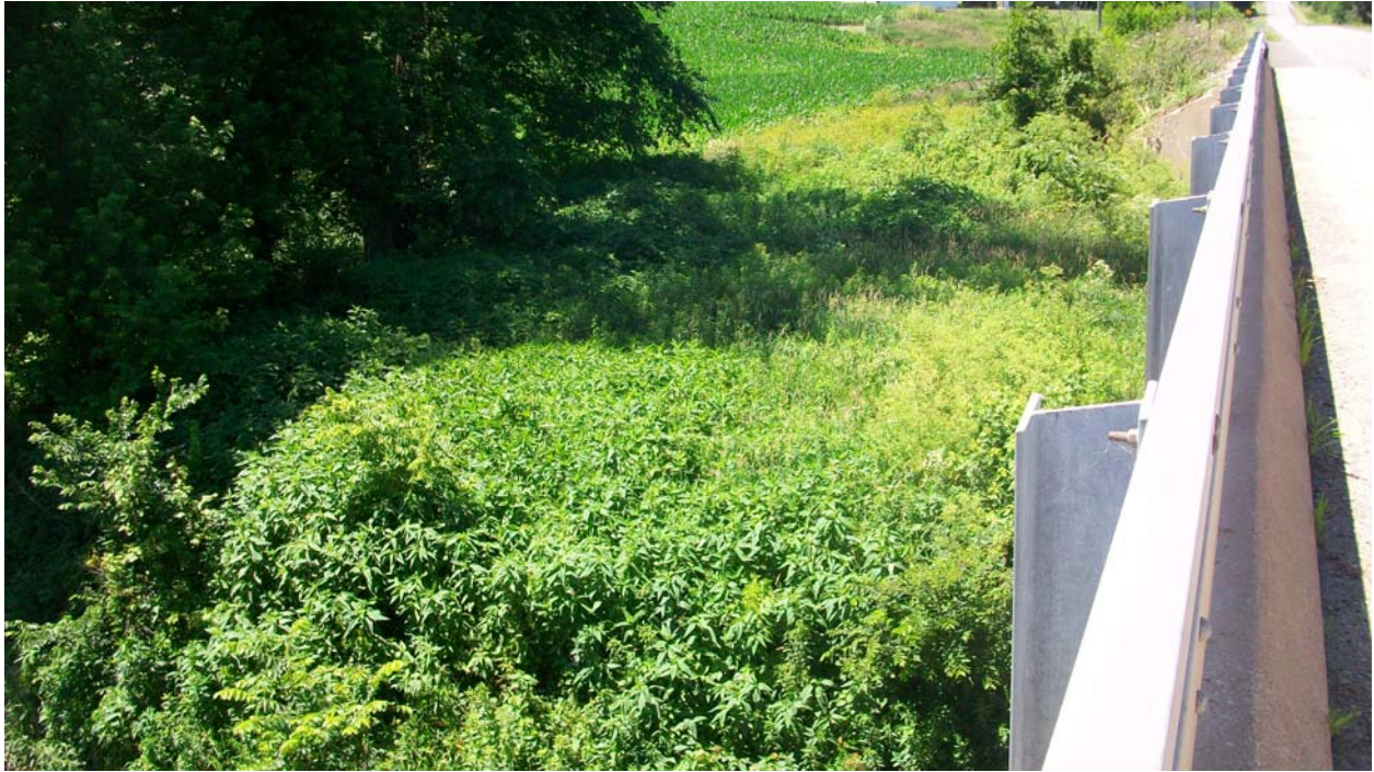
Photo 1 South West Ditch
