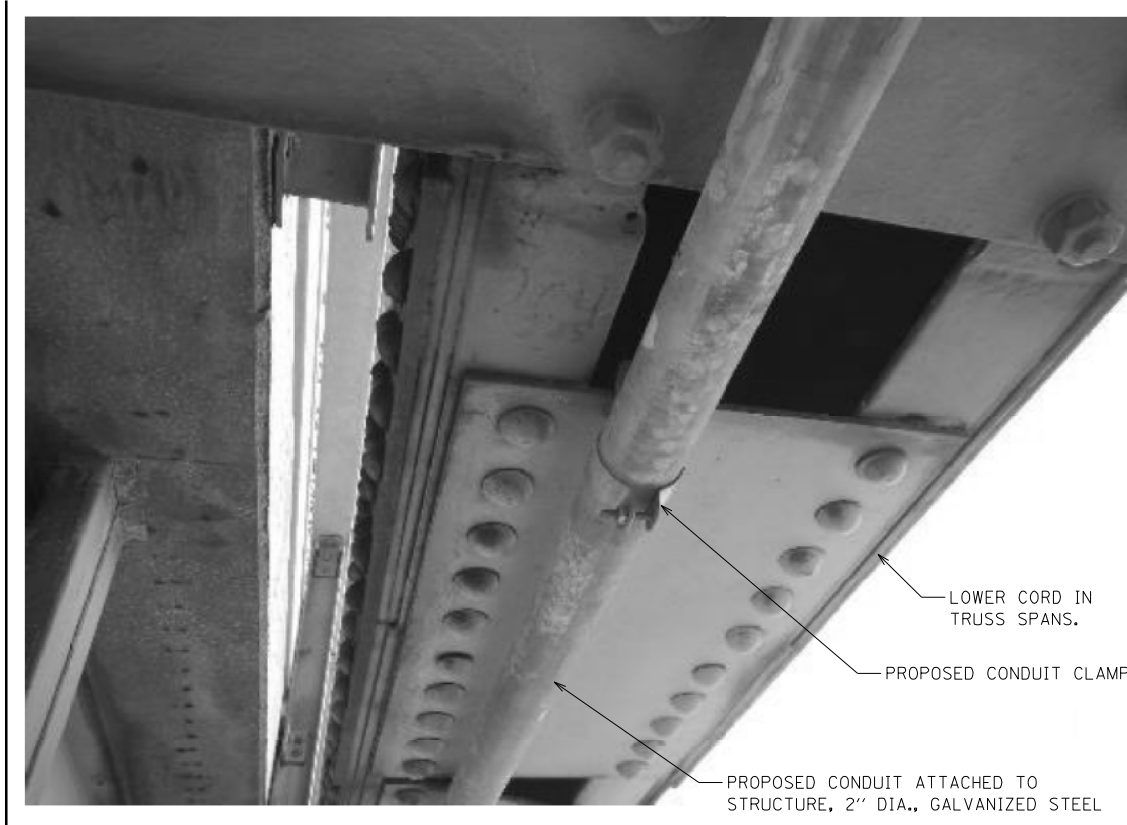
CONDUIT ATTACHED TO STRUCTURE DETAIL
