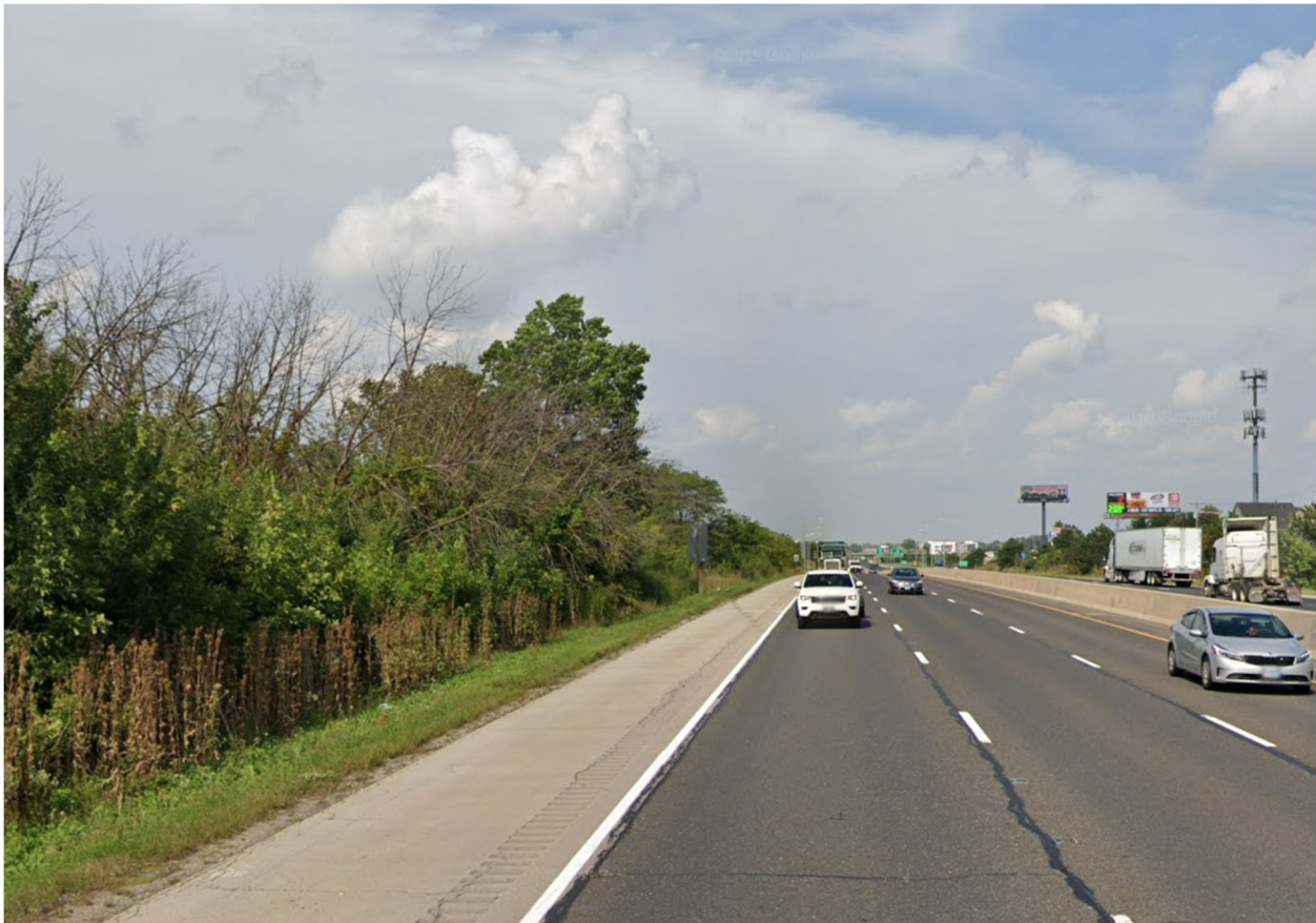
Exhibit 2 – Existing Site Conditions at Proposed Wall Location, Looking north
