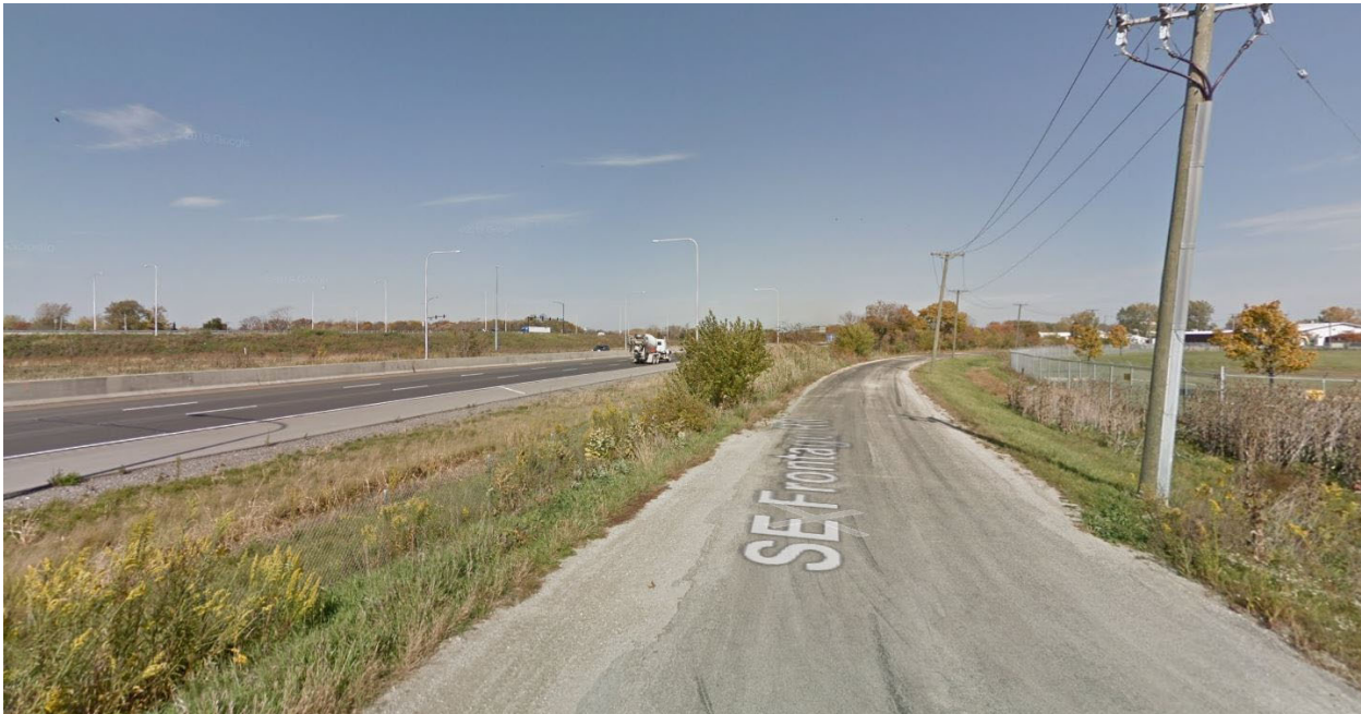
Exhibit 2a – Existing Site Condition, Looking North along SE Frontage Road
