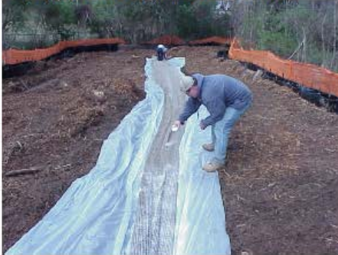
5) Apply Silt Stop (downstream end)
