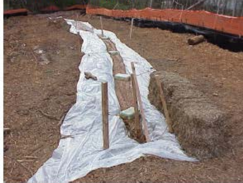
6) Ready for pumping
