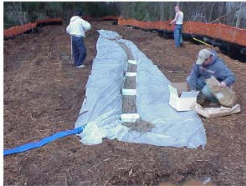
4) Place Floc Logs (upstream end)
