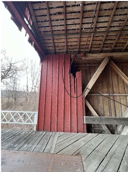
SOUTHWEST INNER PANEL
