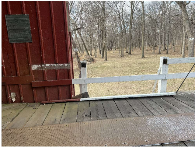
REATTACH TOP RAIL AT NORTHWEST CORNER
