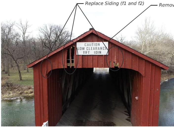
SOUTH FACE OF BRIDGE
