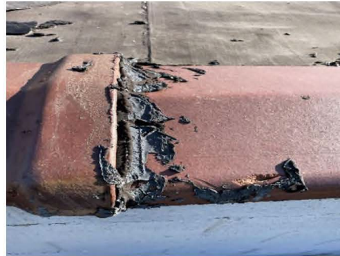
HA-10: Black Roof Coping Tile Sealant
