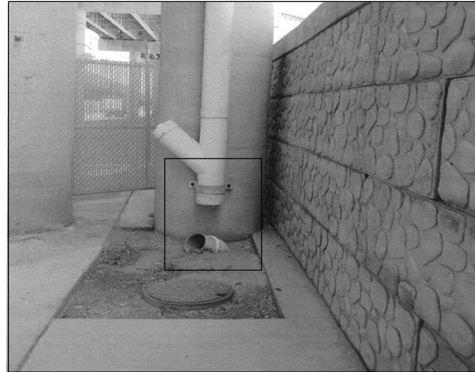
016-1113 PHOTO #2 PIER C5 _ EAST END _ SOUTH FACE
