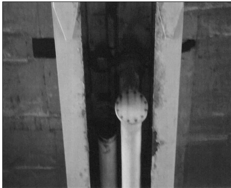
016-1110 PHOTO #4 SPAN 5 _ LOOKING SOUTH
