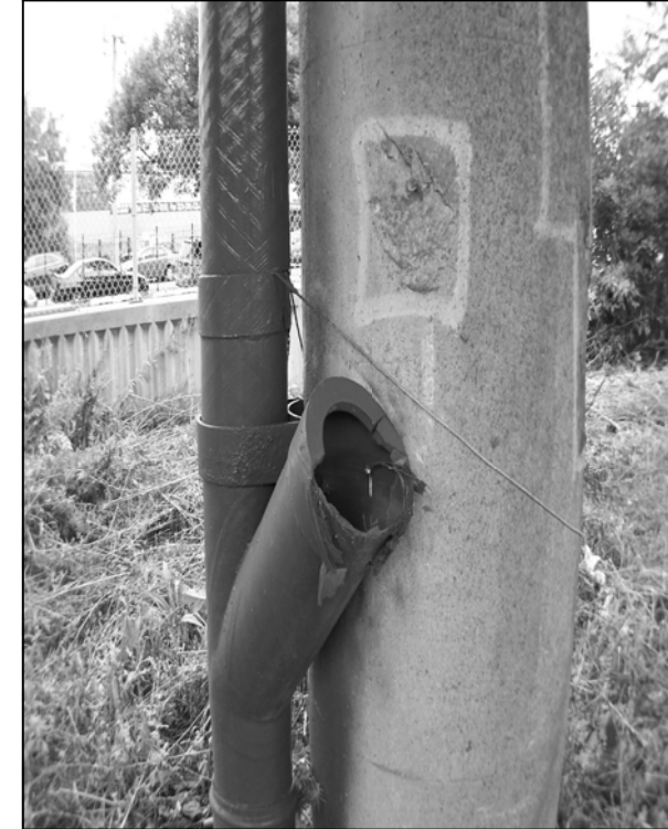
016-1047 PHOTO #2 PIER 27 _ CLOSE UP
