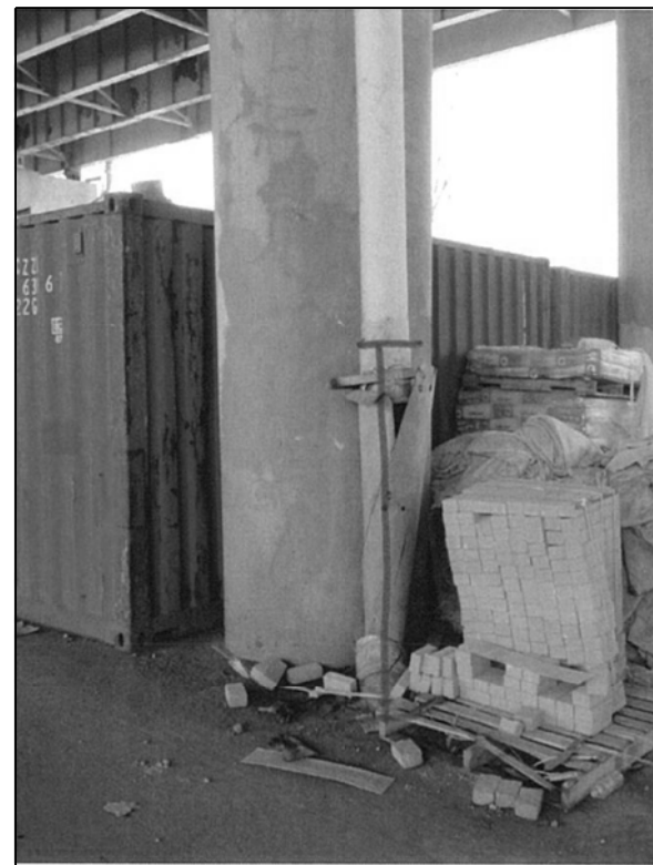
016-1111 PHOTO #5 MAIN LINE PIER 5 _ NORTH FACE
