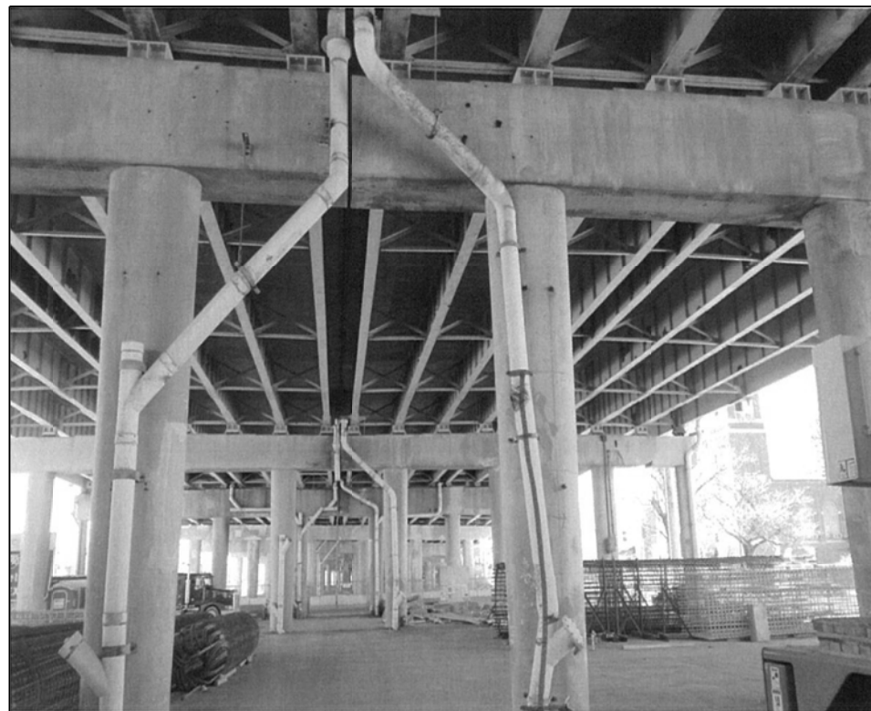
016-1111 PHOTO #4 MAIN LINE PIER 4 _ NORTH FACE
