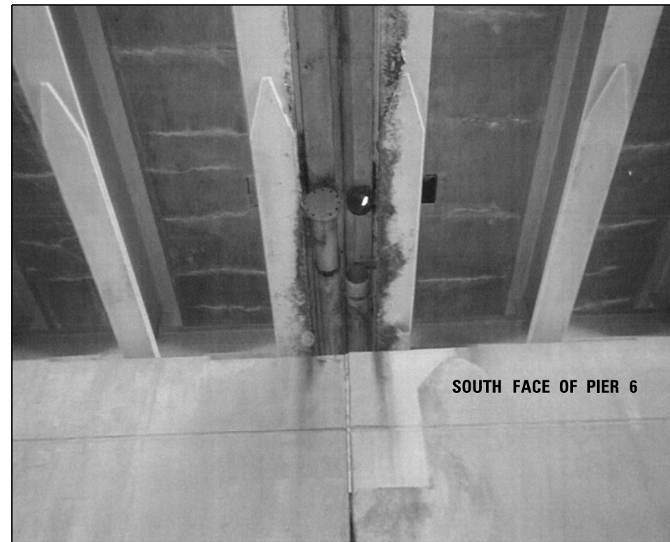
016-1110 PHOTO #5 SPAN 5 _ LOOKING NORTH
