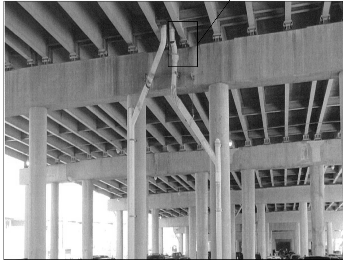
016-0137 - PHOTO #1 SOUTH FACE OF PIER 11
