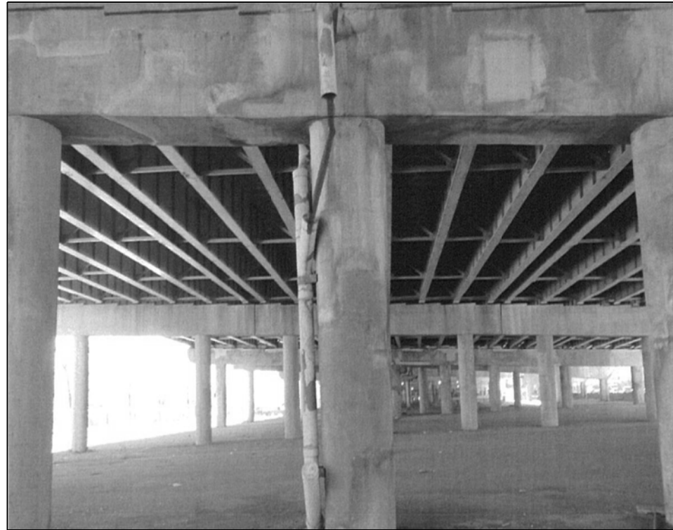
016-1112 PHOTO #1 MAIN LINE PIER 30 _ NORTH FACE
