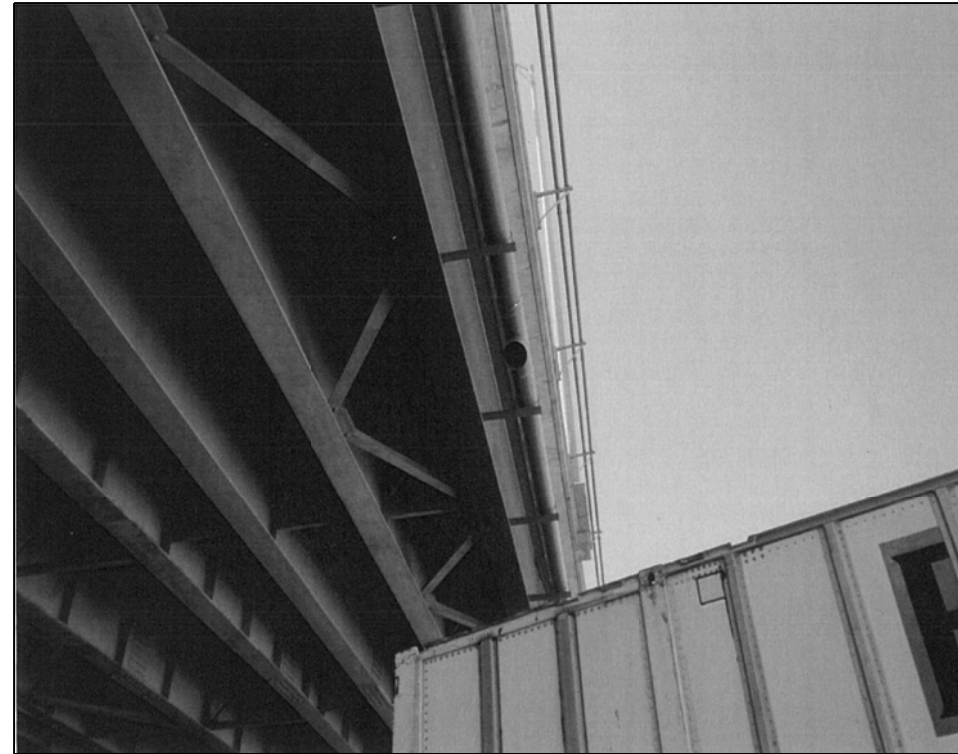
016-1116 PHOTO #2 NORTH FASCIA BEAM - MID SPAN 2
