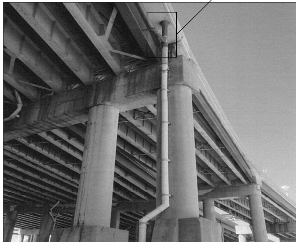
016-1113 PHOTO #3 PIER 1 _ EAST END _ SOUTH FACE
