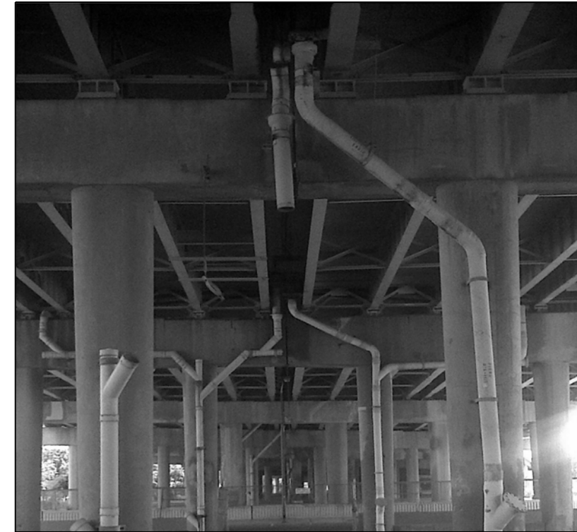
016-1111 PHOTO #3 MAIN LINE PIER 3 _ NORTH FACE
