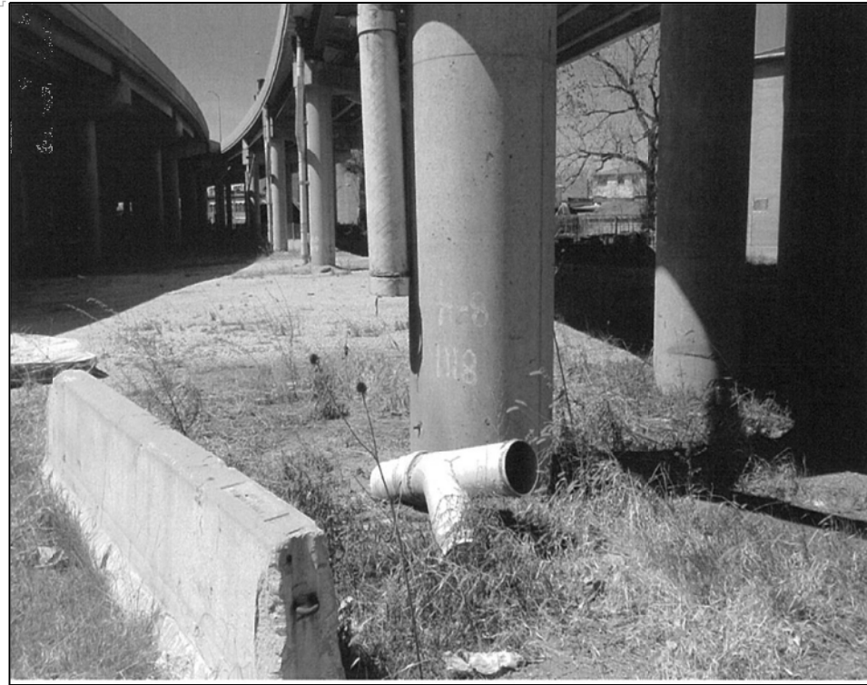
016-1118 PHOTO #1 PIER H8 _ WEST END
