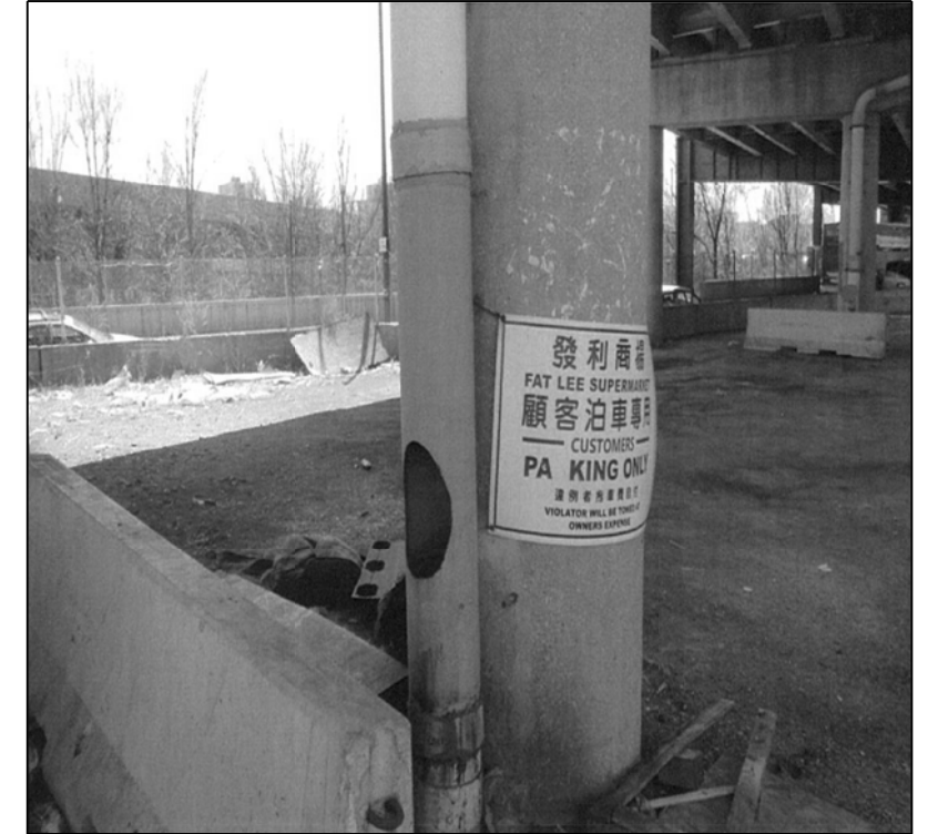
016-1067 PHOTO #3 PIER A7
