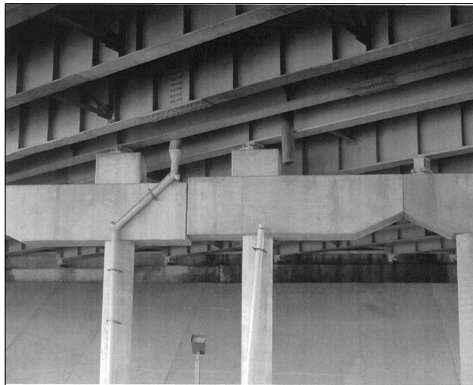
016-0004 AND 016-0005 PHOTO #2 PIER 3 _ WEST FACE
