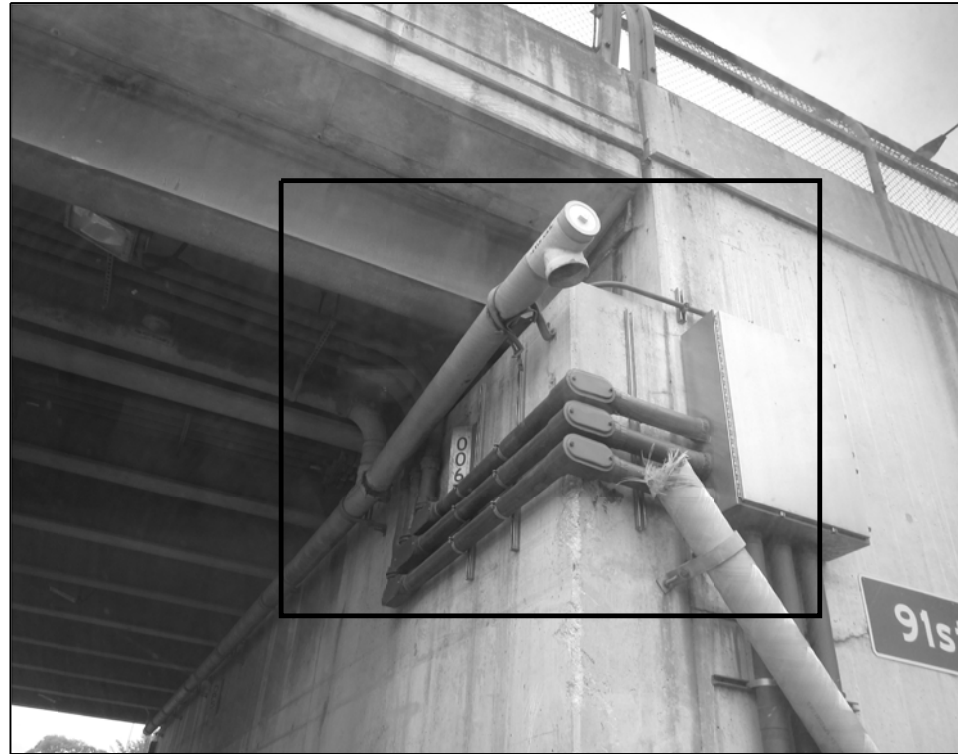
016-1141 PHOTO #1 EAST ABUTMENT _ SOUTH END
