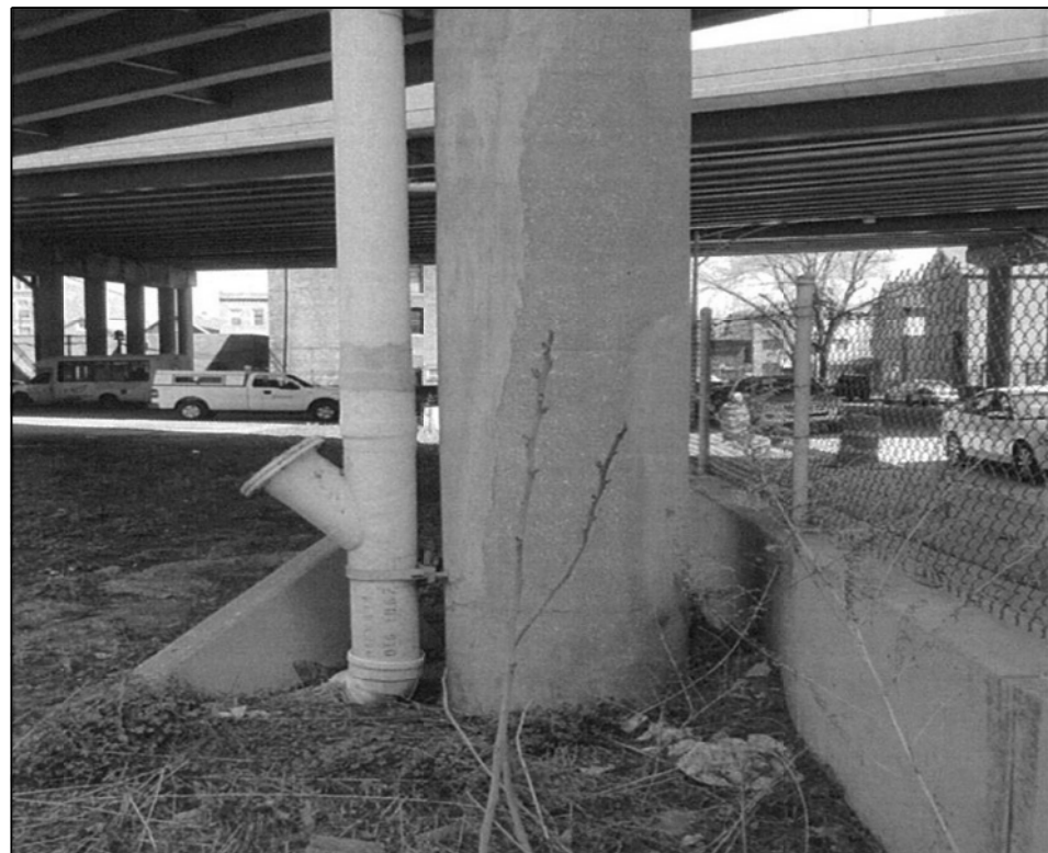
016-1067 PHOTO #4 SPAN A14
