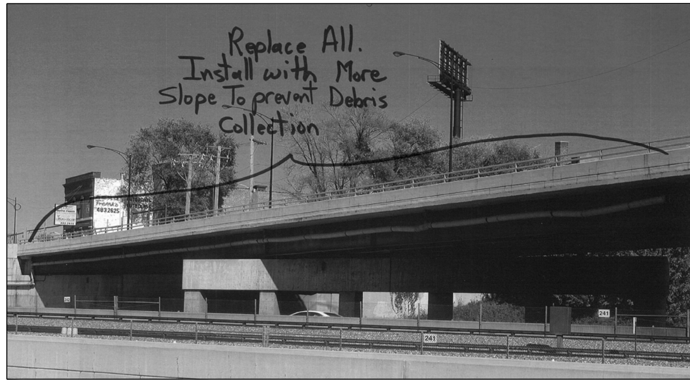
016-1007 PHOTO #4 SECTION OVER DAN RYAN NB LANES _ LOOKING EAST
