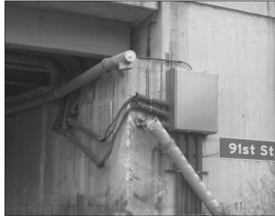
016-1141 PHOTO #2 EAST ABUTMENT _ SOUTH END
