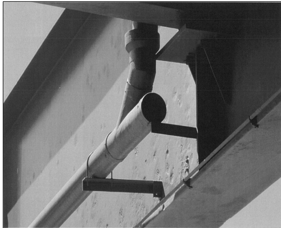
016-1118 PHOTO #3 PIER H2 _ SOUTH FACE
