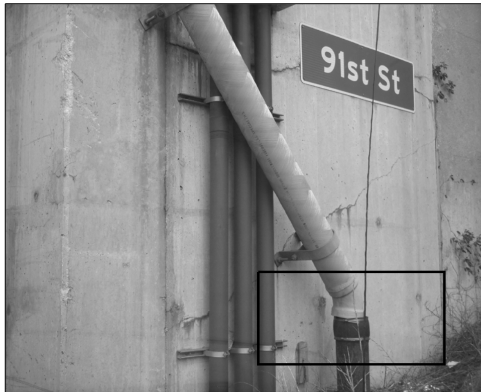
016-1141 PHOTO #3 EAST ABUTMENT _ SOUTH END
