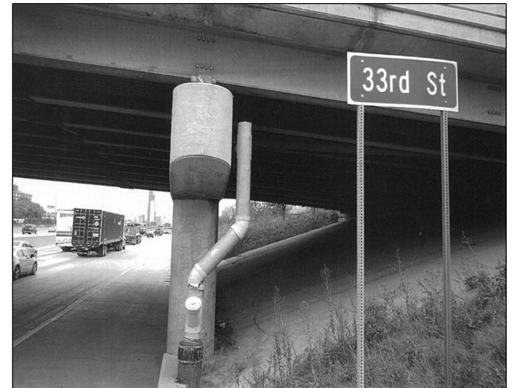
016-1158 PHOTO # PIER 6 _ SOUTH END
