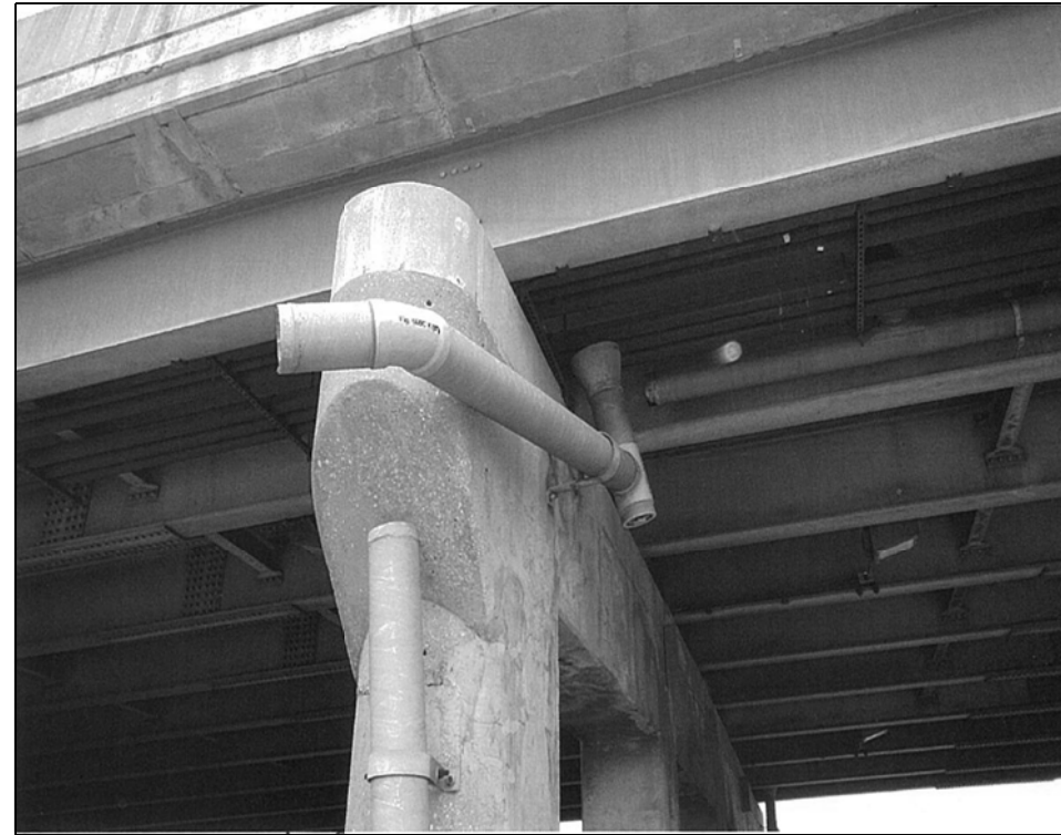
016-1151 PHOTO #2 PIER 1 _ SOUTH END
