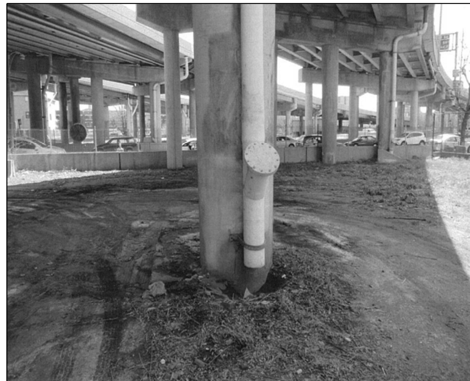
016-1067 PHOTO #5 SPAN A15
