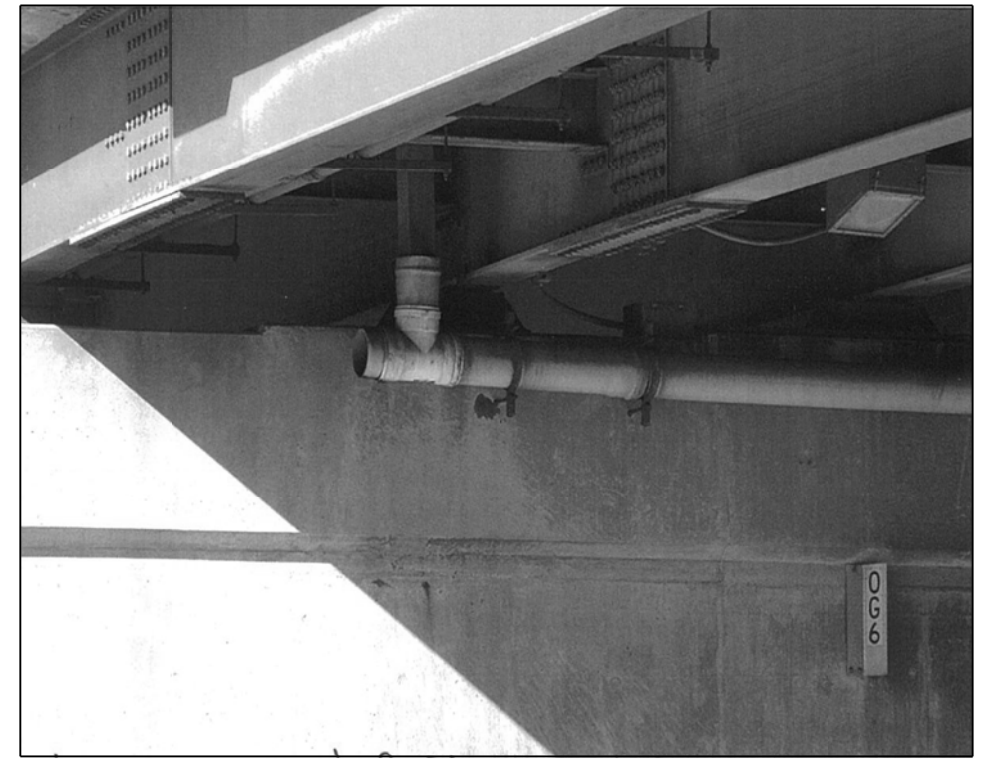
016-1142 PHOTO #1 PIER 2 - EAST FACE - SOUTH END
