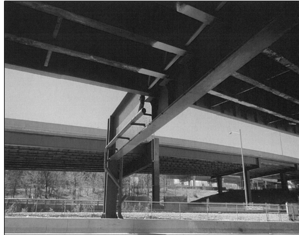
016-1118 PHOTO #2 PIER H2 _ SOUTH FACE
