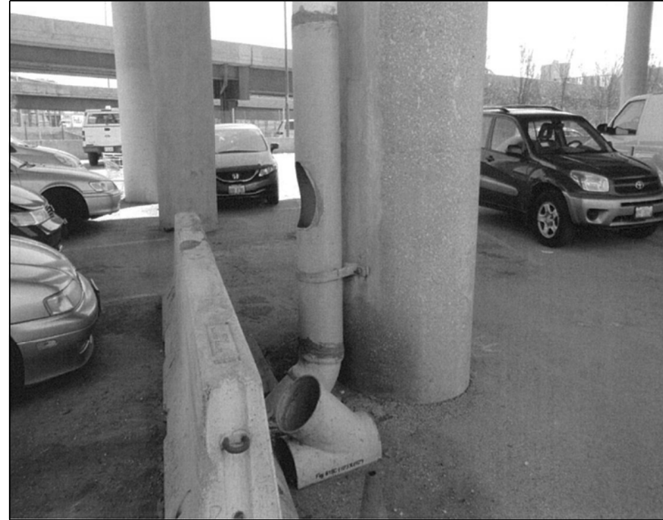
016-1067 PHOTO #2 PIER A6
