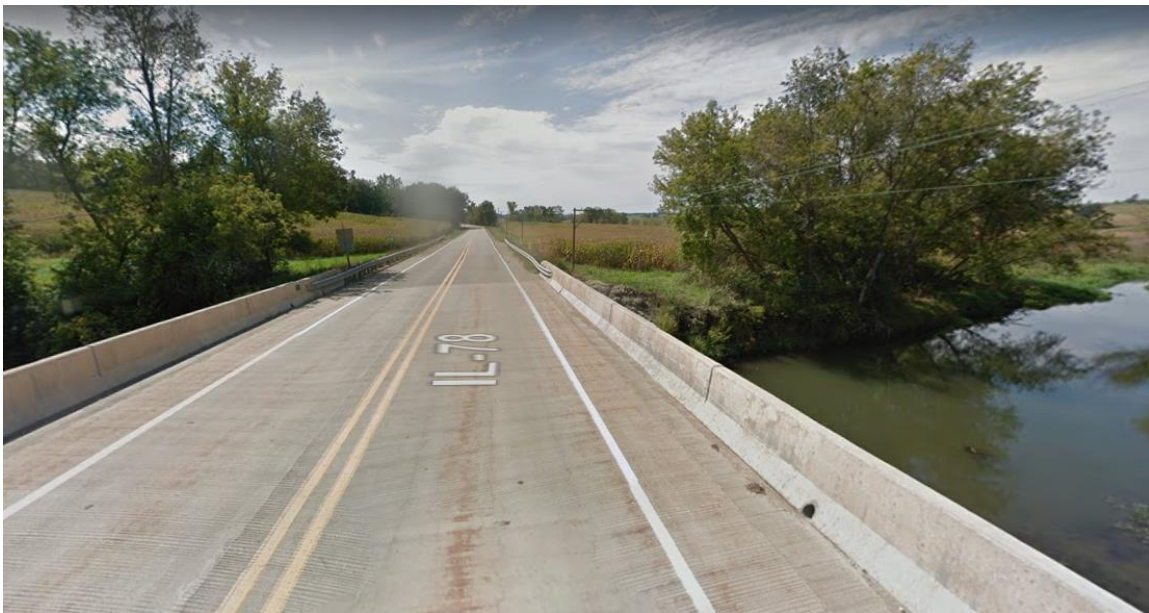
Exhibit 2b: Structure 043-0040, looking south from bridge
