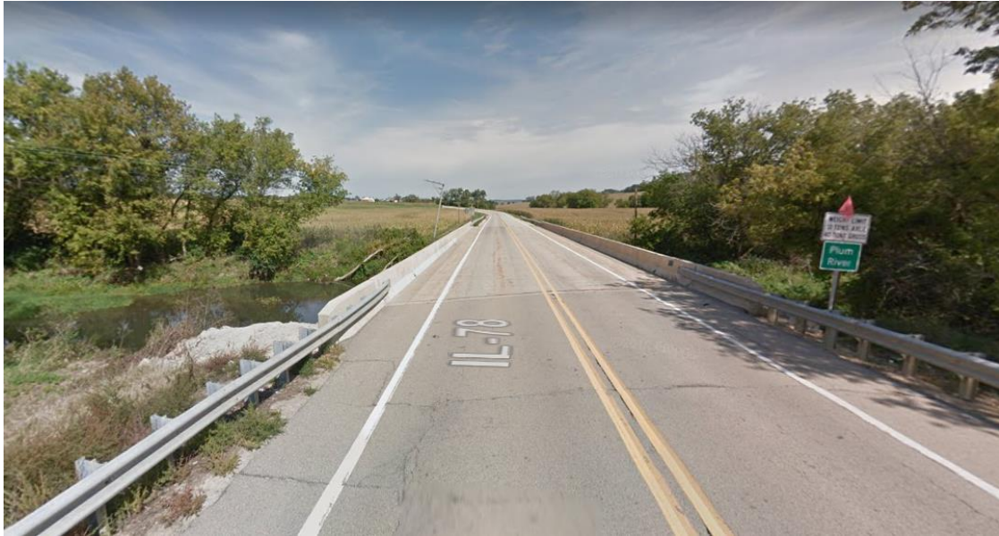
Exhibit 2a: Structure 043-0040, looking north from bridge
