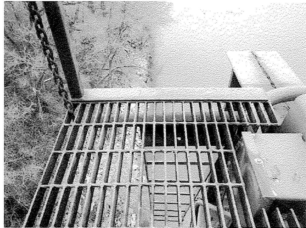
ITEM 677 Span 9, LOS (Catwalk) See Note A
