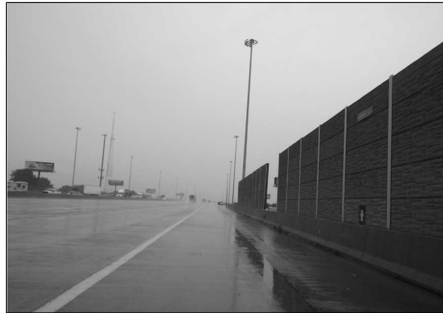
PRECAST CONCRETE WALL REPLACE 23'-4" OF WALL
