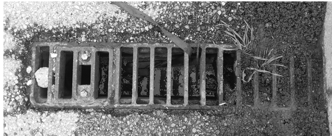
(A) CLEANING EXISTING DRAINAGE SCUPPERS
