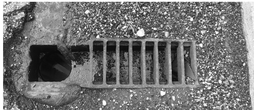
(B) CLEANING AND REPAIR DRAINAGE SCUPPERS SN 050-0164 NORTHBOUND LT.
