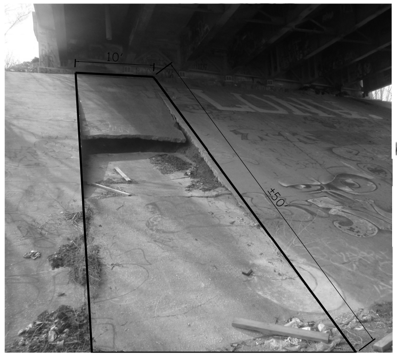
SLOPE WALL REPAIR AREA
