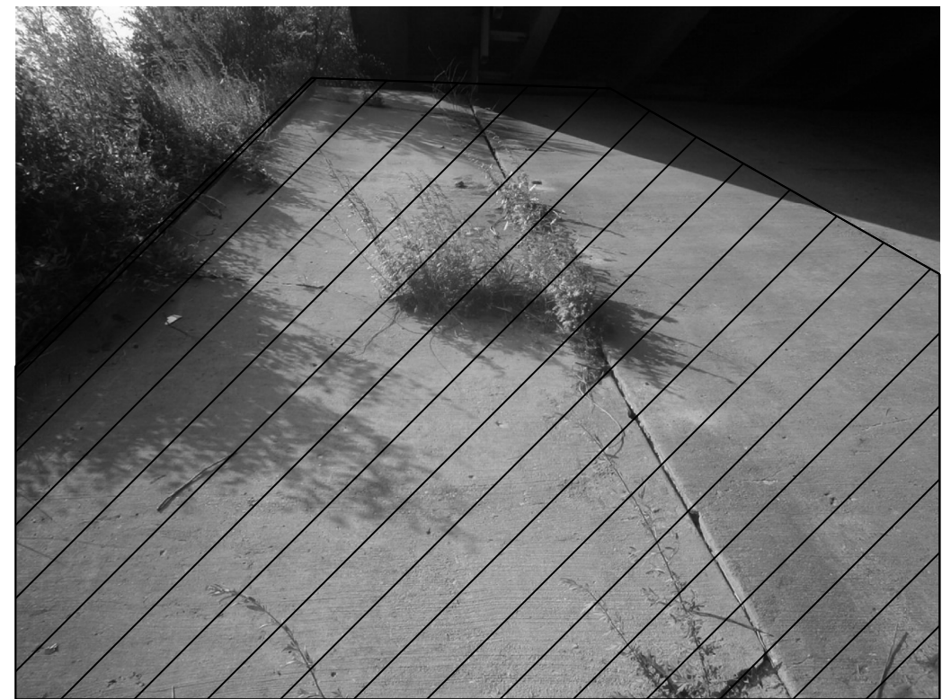
SLOPE WALL REPAIR AREA SOUTHEAST
