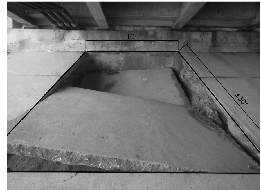
SLOPE WALL REPAIR AREA
