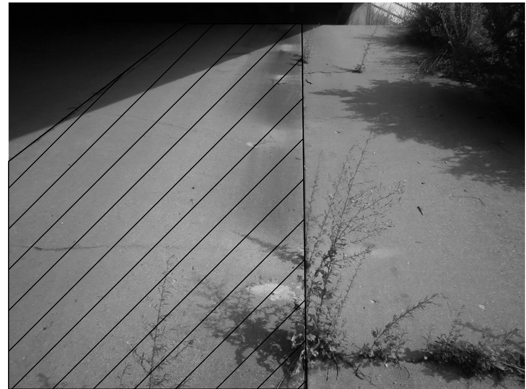
SLOPE WALL REPAIR AREA NORTHEAST
