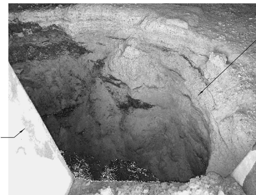
PHOTO 2 Inside East Abutment Vault
