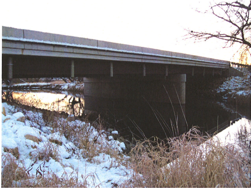
Thorndale Ave Upstream Face
