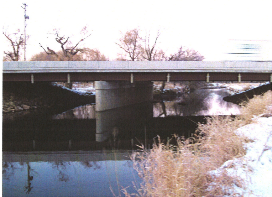
Thorndale Avenue Downstream Face
