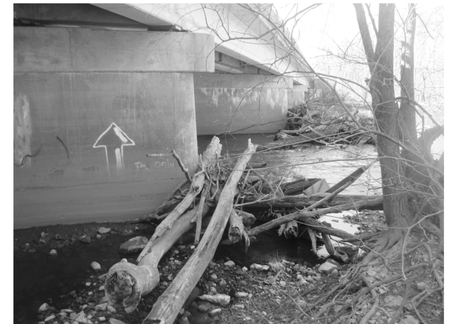
DEBRIS REMOVAL NEAR PIER 3
