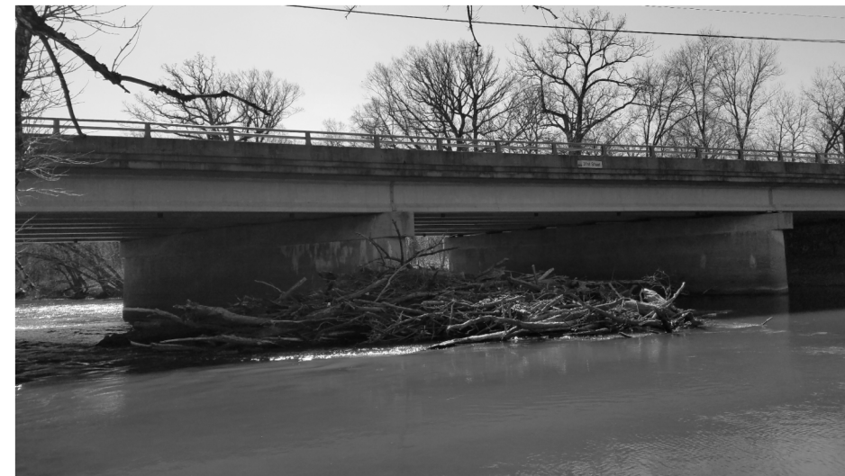
DEBRIS REMOVAL NEAR PIER 2
