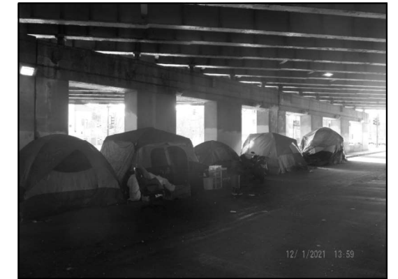
EXISTING LIGHTING: PIER 1 (Looking Southwest)
