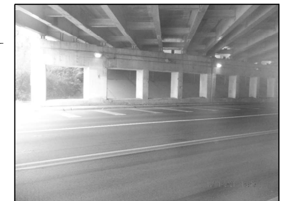
EXISTING LIGHTING: PIER 2 (Looking Northwest)
