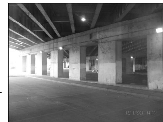
EXISTING LIGHTING: PIER 2 (Looking Northwest)
