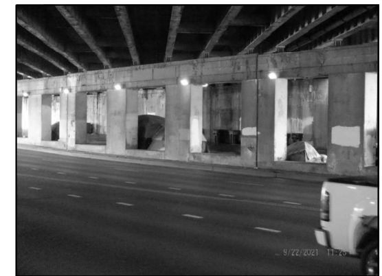
EXISTING LIGHTING: PIER 1 (Looking Northwest)
