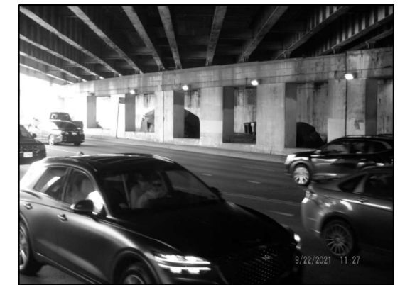
EXISTING LIGHTING: PIER 1 (Looking Northwest)
