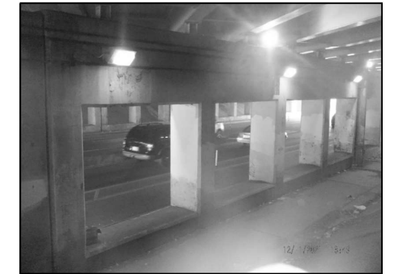
EXISTING LIGHTING: PIER 1 (Looking Northwest)
