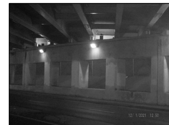
EXISTING LIGHTING: PIER 1 (Looking Northeast)
