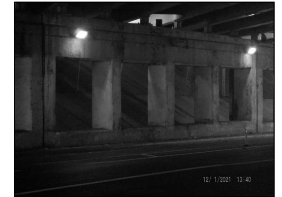
EXISTING LIGHTING: PIER 2 (Looking Northwest)
