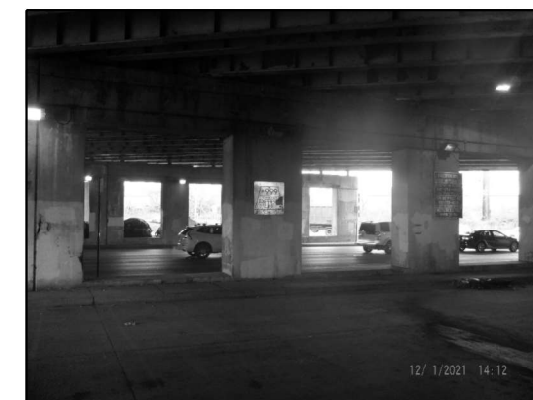
EXISTING LIGHTING: PIER 2 (Looking Northwest)
