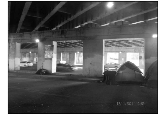
EXISTING LIGHTING: PIER 1 (Looking Southeast)
