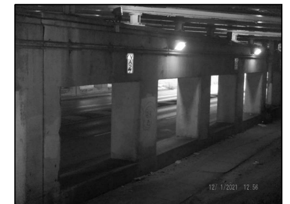
EXISTING LIGHTING: PIER 2 (Looking Northeast)
