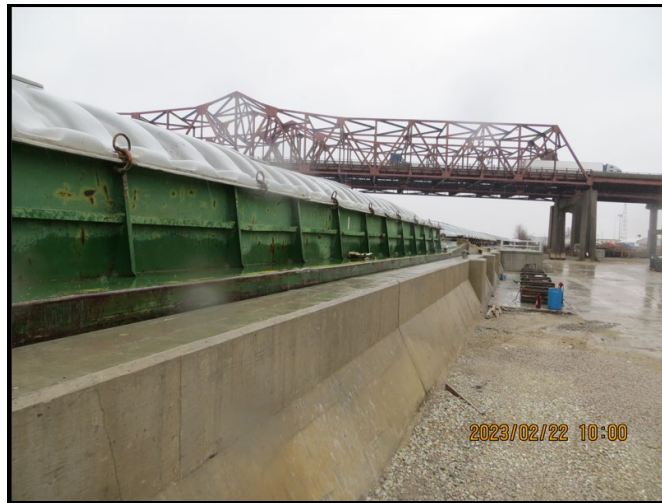
Photo 1. General photo of floodwall (at Ozinga property), looking south.
