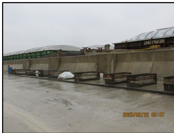
Photo 2. Close up photo of floodwall (at Ozinga property), looking northeast.
