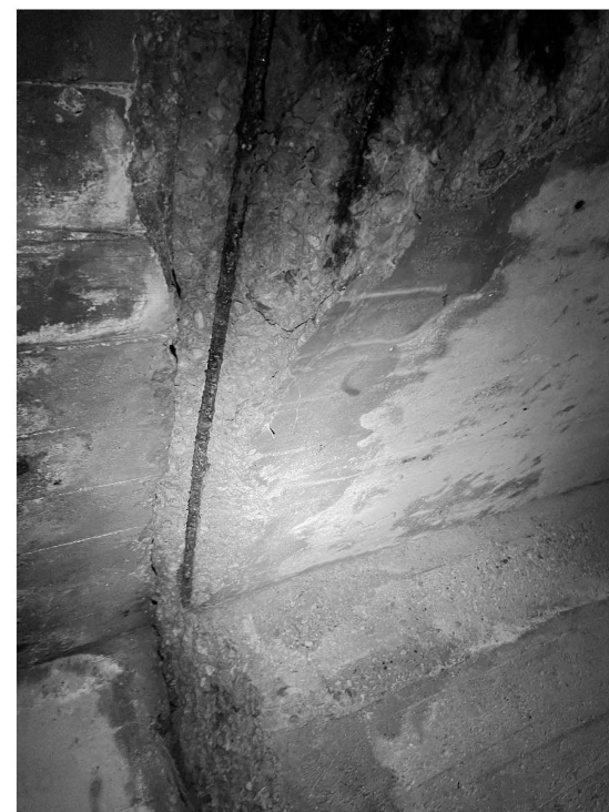
Typical Condition - Culvert Sta. 00+16
