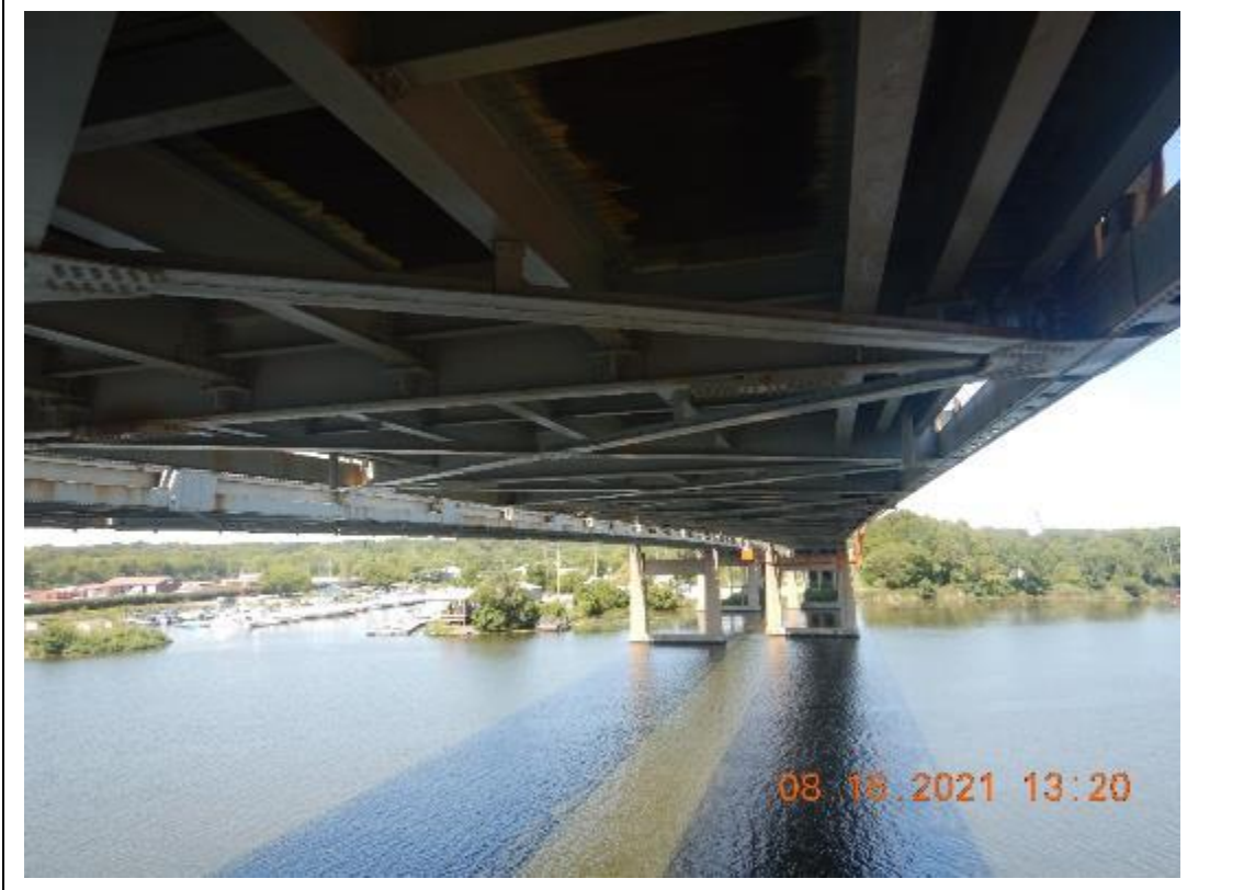
PHOTO 1 SPAN 5, LOOKING NORTH
