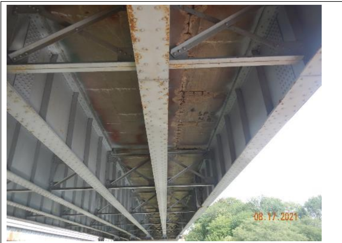
PHOTO 8 SPAN 3, LOOKING NORTH
