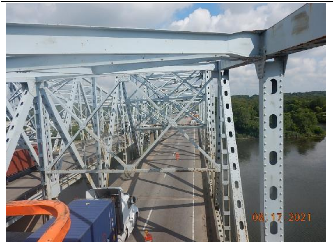
PHOTO 4 SPAN 5, LOOKING NORTH
