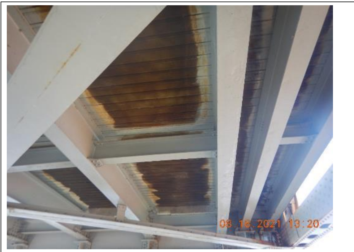
PHOTO 10 SPAN 5, LOOKING SOUTH
