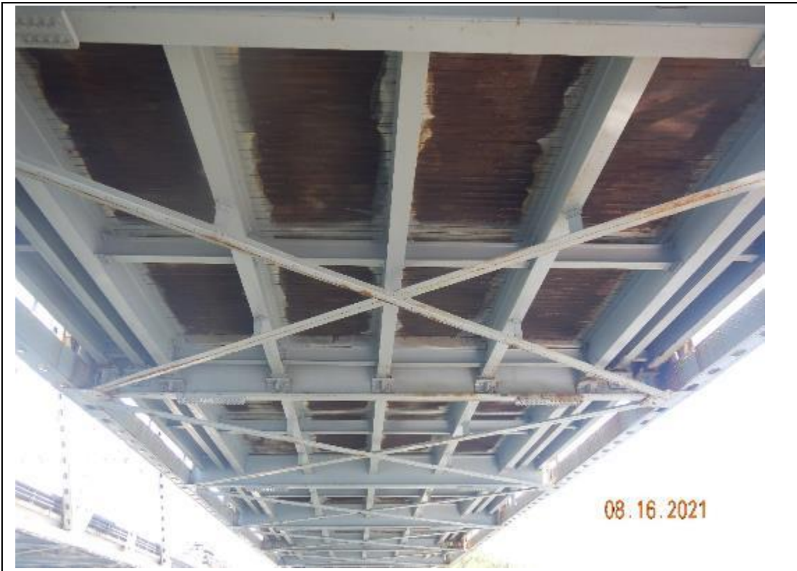
PHOTO 9 SPAN 4, LOOKING NORTH
