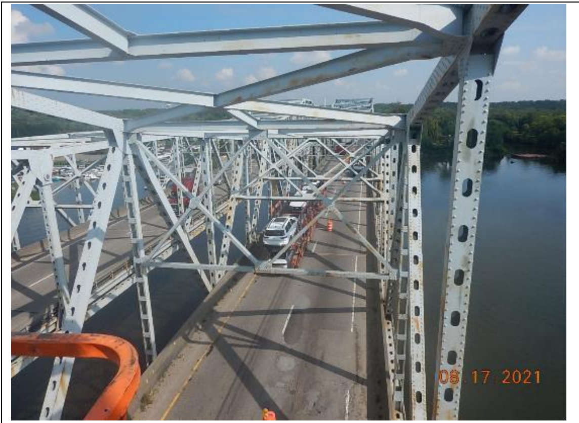
PHOTO 3 SPAN 6, LOOKING NORTH
