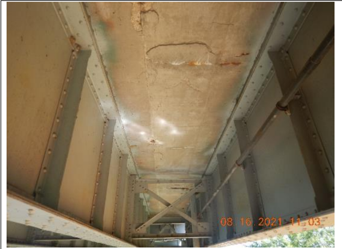
PHOTO 7 SPAN 7, LOOKING NORTH
