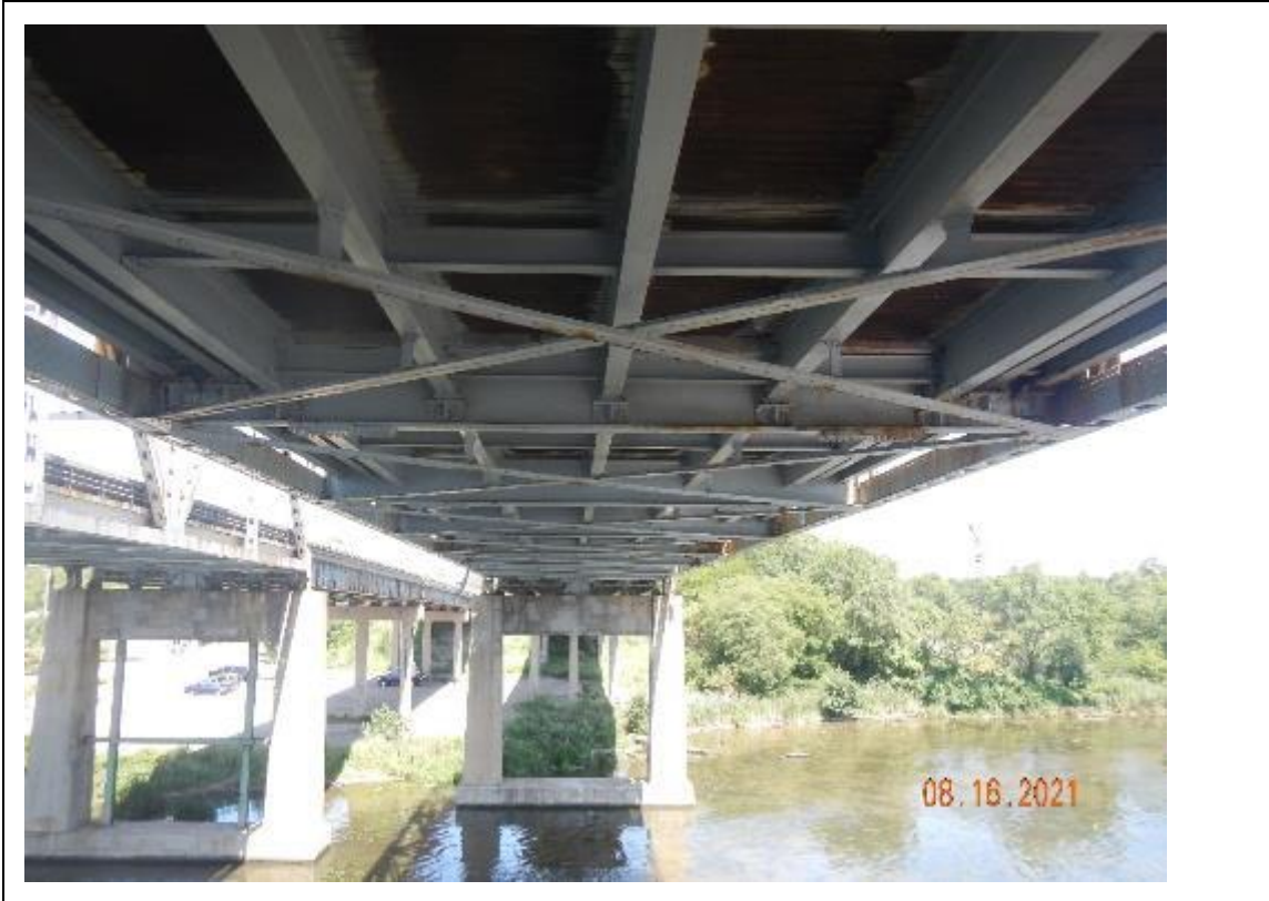
PHOTO 2 SPAN 4, LOOKING NORTH
